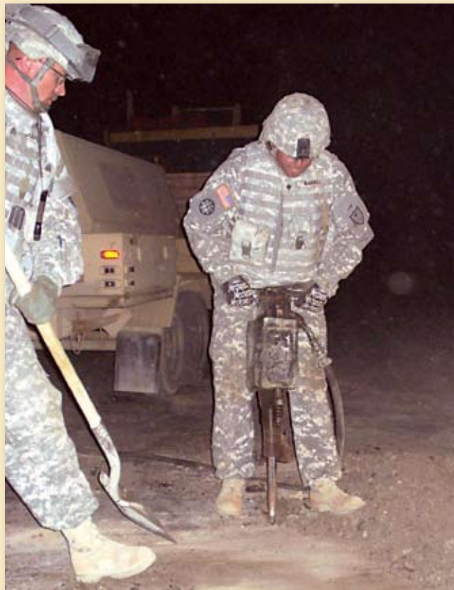
Engineers finish filling a crater in a road.
