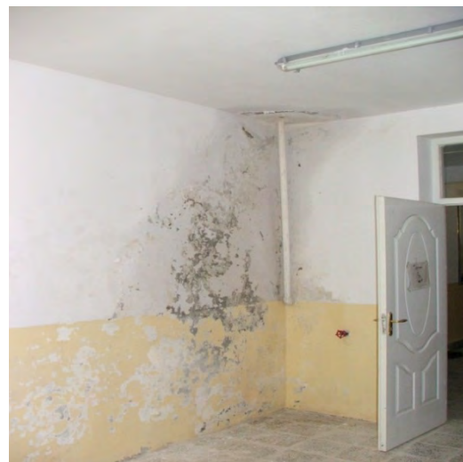
Photo 2 - Leaky Roof Damages Ceilings and Walls
