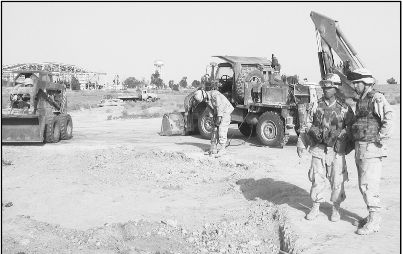
Soldiers from the 887th Engineer Company use a small emplacement excavator (SEE) and a Bobcat® to repair a crater in an airfield in northern Iraq.
