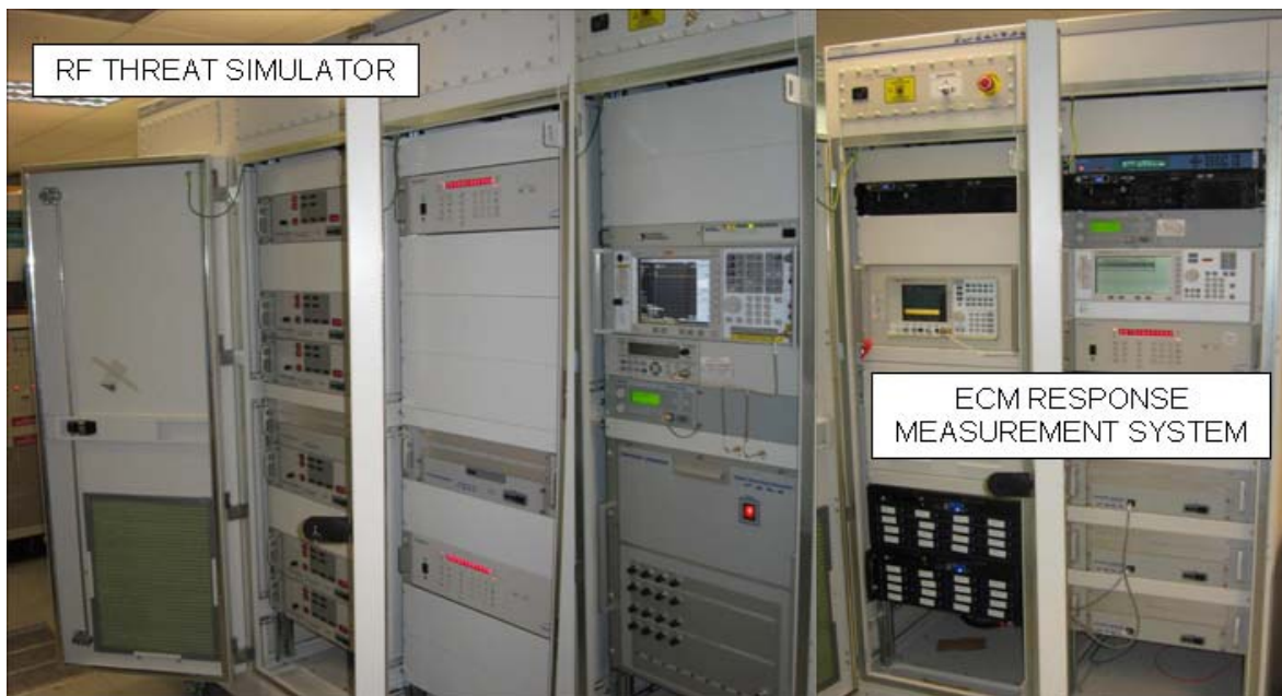
Figure 6-3: RF Threat Emitter Simulator and EA/ECM Signal Measurement System – (BAE SYSTEMS Photograph).
