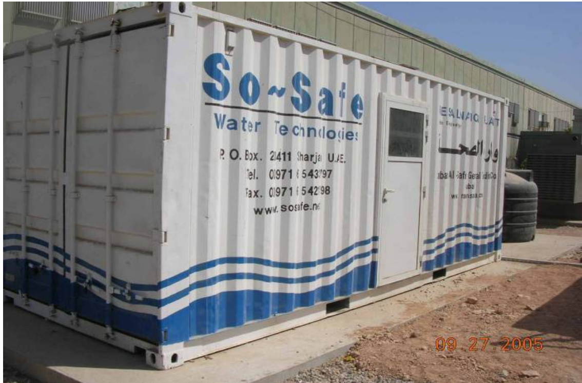
Site Photo 3. Exterior Reverse Osmosis Containerized Unit (Photo courtesy of the USACE QAR)
