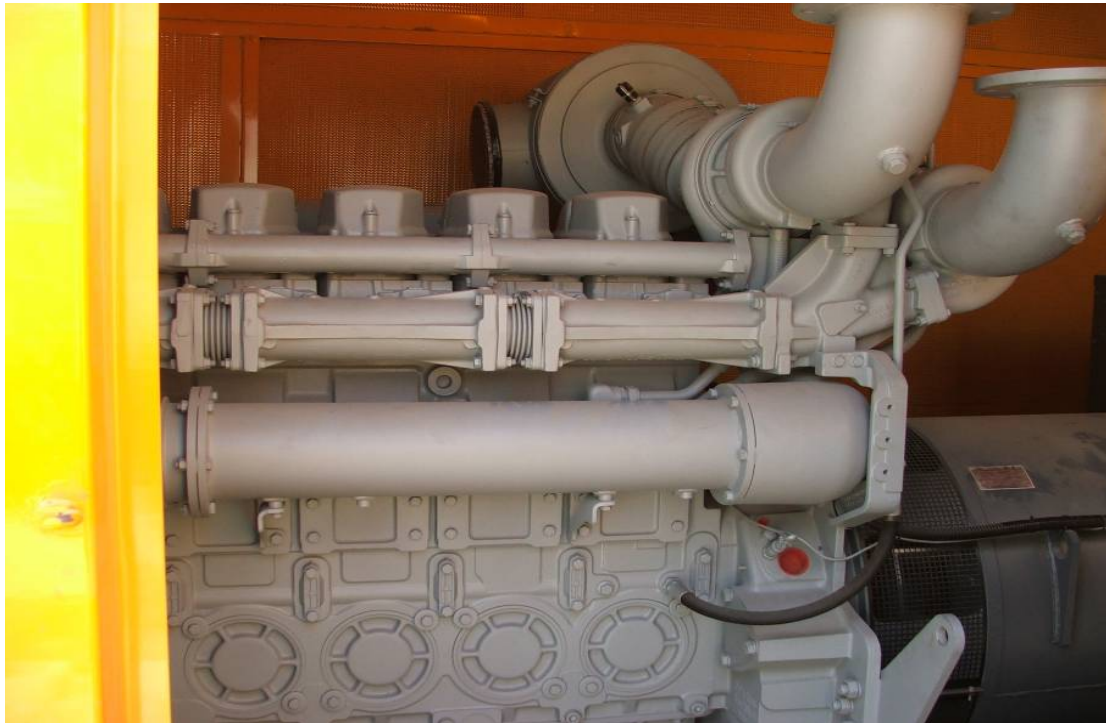
Site Photo 5. Generator Motor and Alternator
