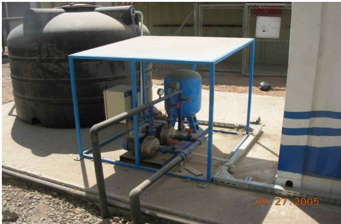
Site Photo 4. Raw Water Tanks and High Pressure Feed Pumps (Photo courtesy of the USACE QAR)
