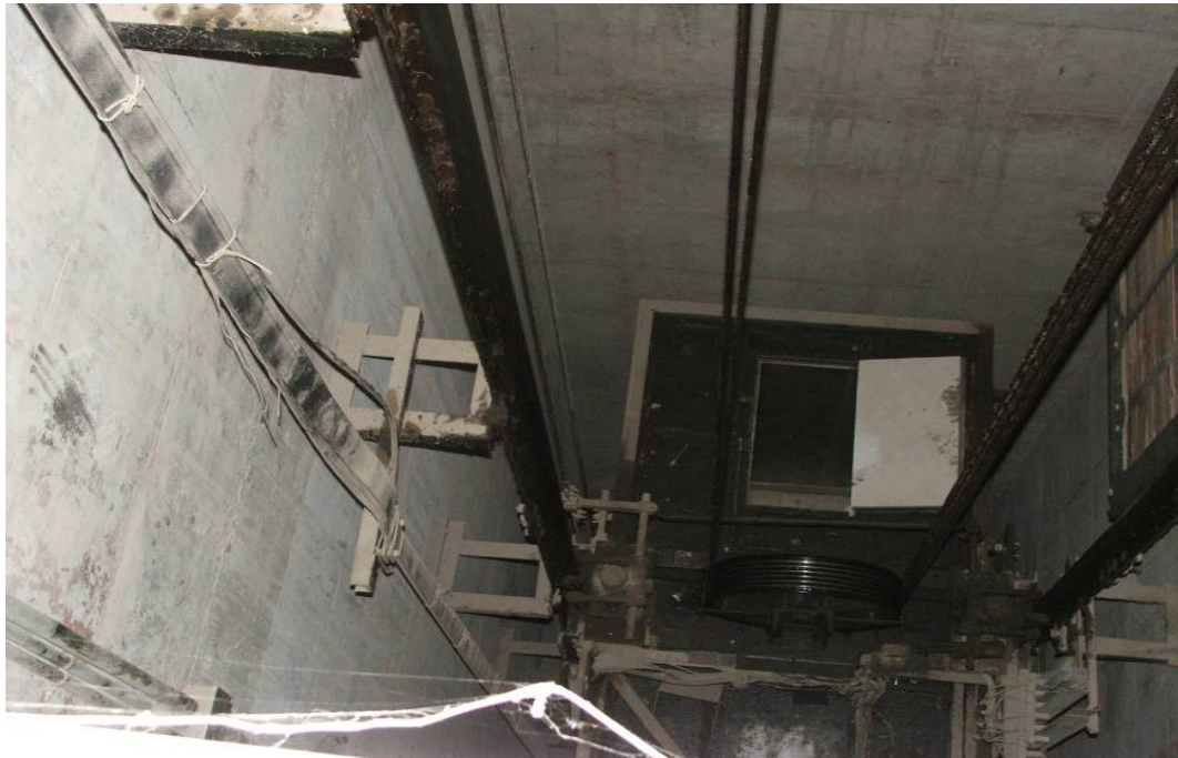
Site Photo 9. Inside of the Elevator Shaft
