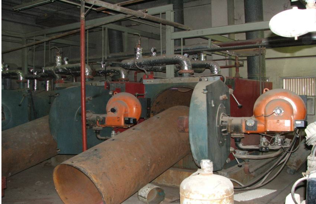
Site Photo 7. Partially Dismantled Boiler Unit
