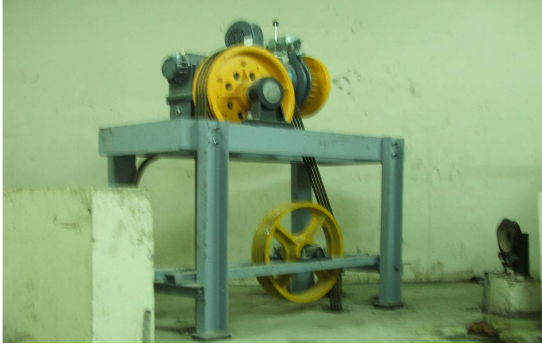
Site Photo 8. Newly Installed Motor for the Elevator Unit
