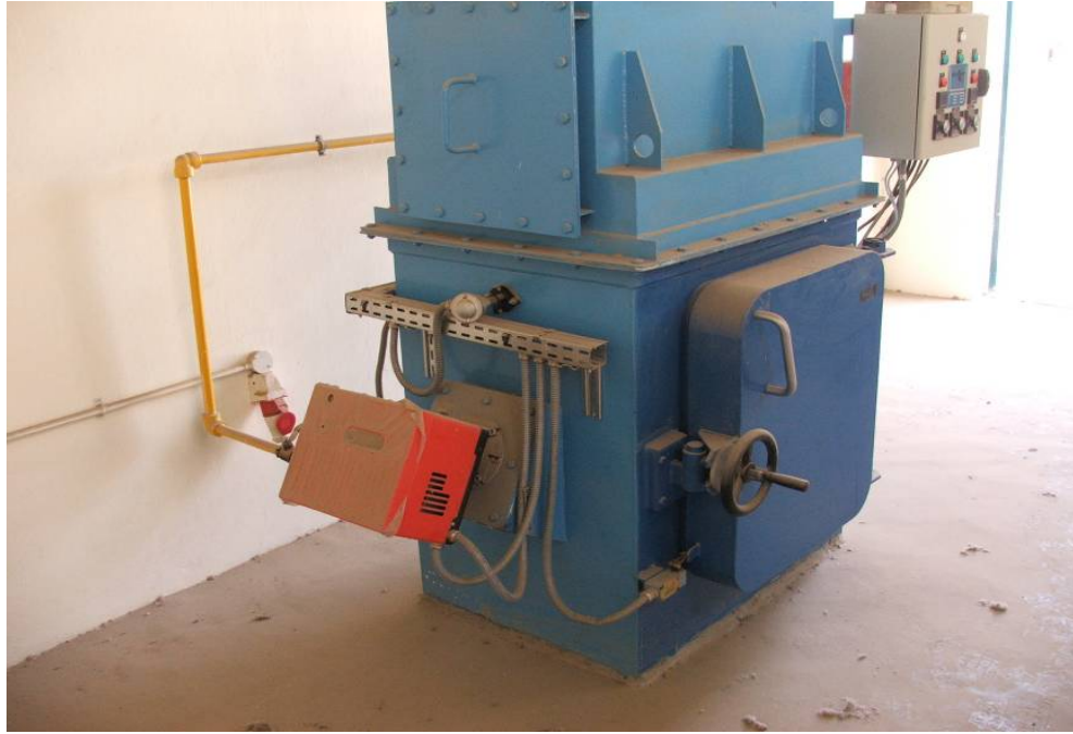
Site Photo 2. Installed Incinerator and Unit Controls
