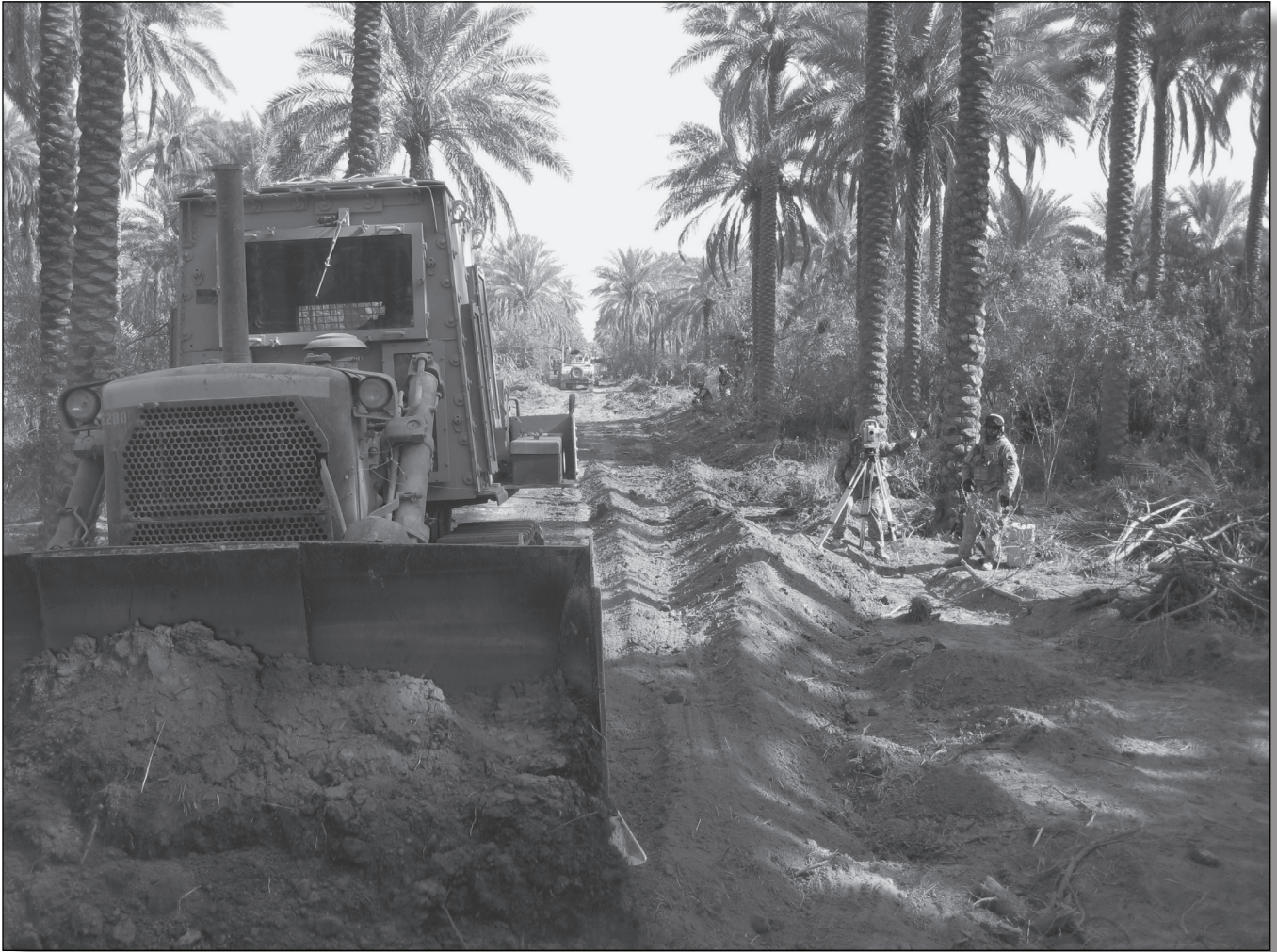
Engineers clear and grub a road during construction operations.
