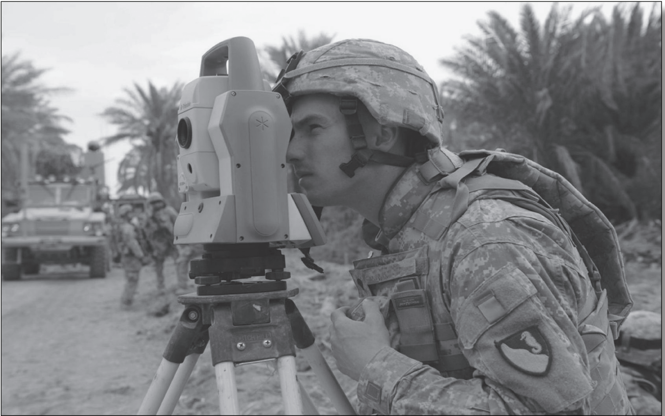
A 5th Engineer Battalion survey team sights in a road during construction operations.
