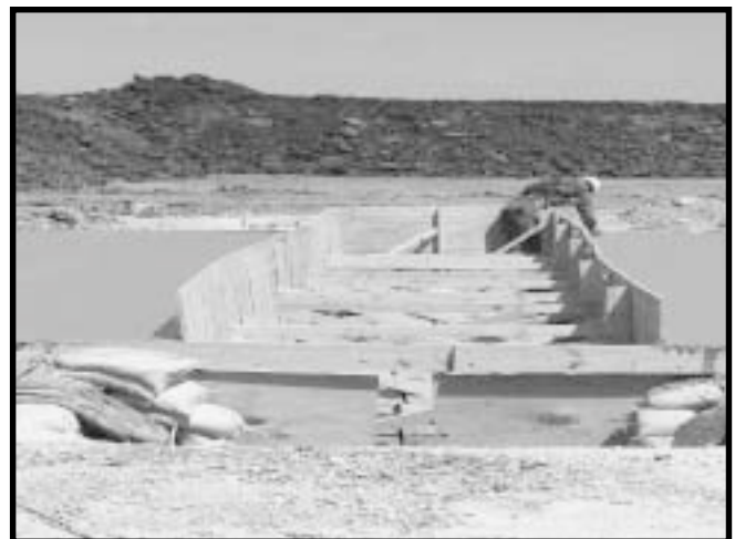
Figure 1. These forms were poorly constructed and not inspected. Notice the blowing and waving effect.
