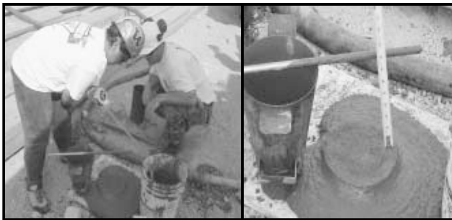
Figure 3. County inspectors assist the unit QC representative in conducting a “slump” test for a grout fill on a CMU block wall. The slump was to be about 8 inches.
