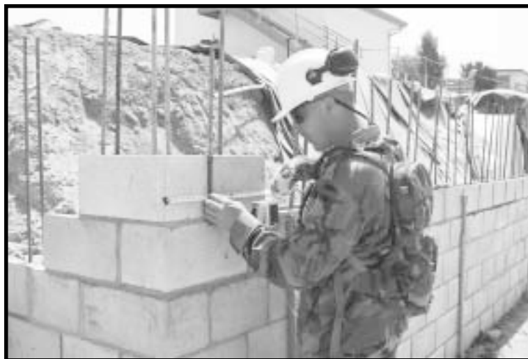
Figure 2. This QC NCO ensures that the CMU wall and block are properly located and measured/cut for placement.
