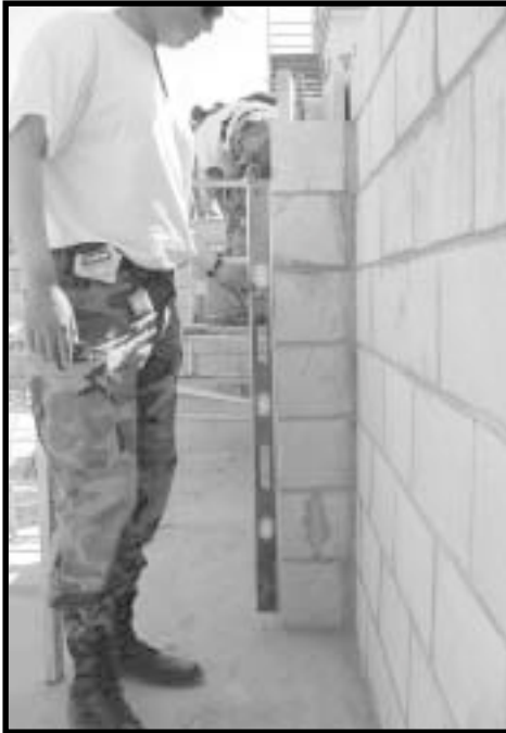
Figure 5. This pilaster is “out of plumb” by 1 1/4 inch on the seventh course, the second course CMU block is cut, and the mortar joints are sloppy.
