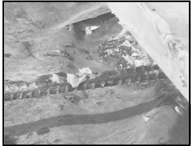
Figure 6. The grease on this rebar will not allow the concrete to adhere around the reinforcement as it should. More care should be taken when lubricating forms.
