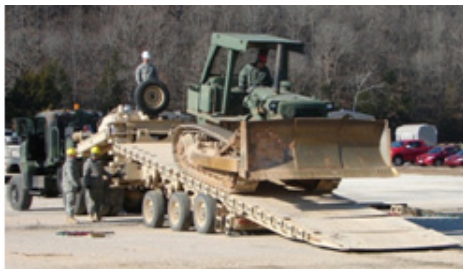
Figure 33: JRaDS 34T loading demo with D7G bulldozer over plywood dunnage.
