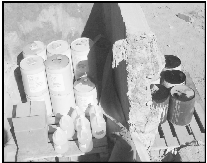
The leaking containers at right should be in the plastic-lined pit at left. Unopened containers at left should be stored elsewhere.
