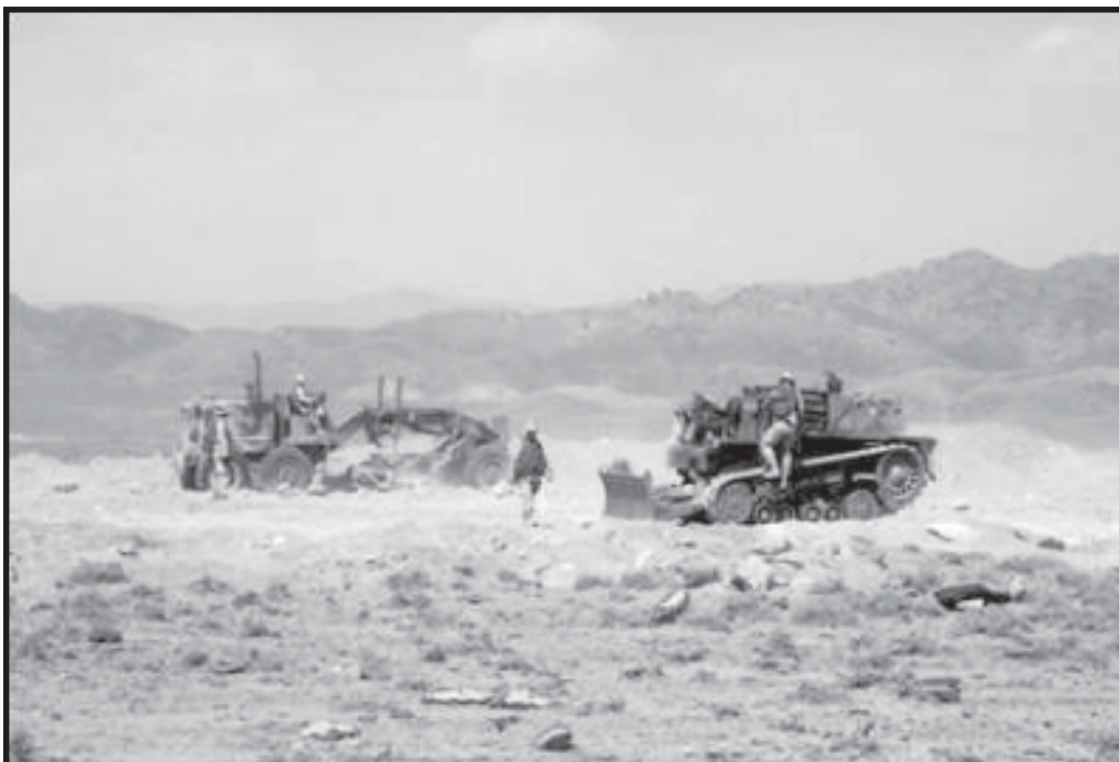
ALZ construction 12 hours after the airborne operation
