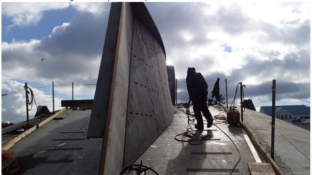
Sally Ride Block 6 Stern – Ballast Tank 4P was blasted and inspected. No defects noted. Surface
