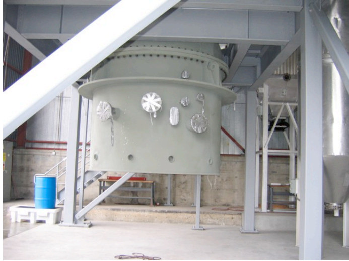
Figure 10. Reactor Suspended from Superstructure
