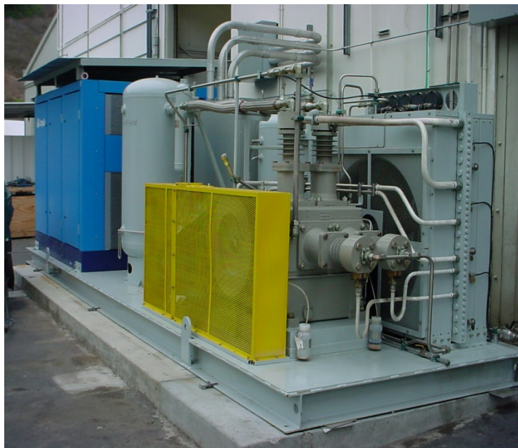
Figure 3. High Pressure Air Compressor
