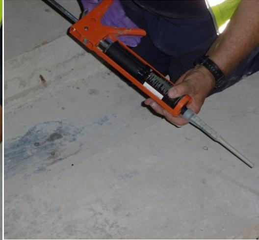
Figure 12. Two-part epoxy-mixing caulking gun.
