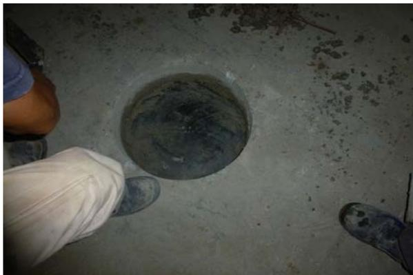
Figure 9. 16 in. diameter core hole cut to expose steel EMS for testing.
