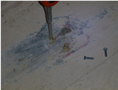
Figure 13. Close-up photo of epoxy injection.
