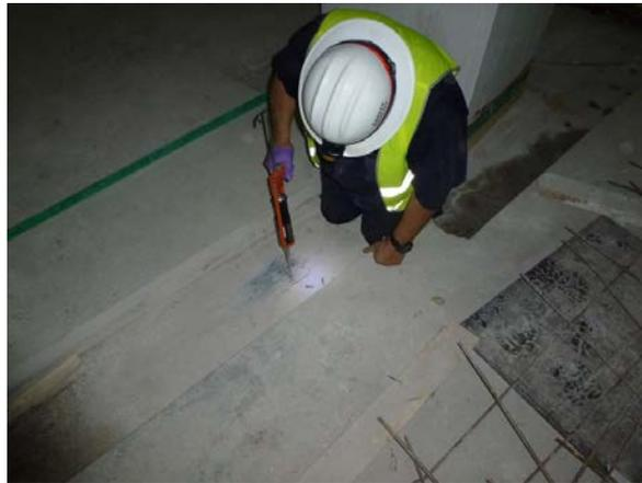
Figure 8. Existing trough in concrete liner over EMS steel plate.
