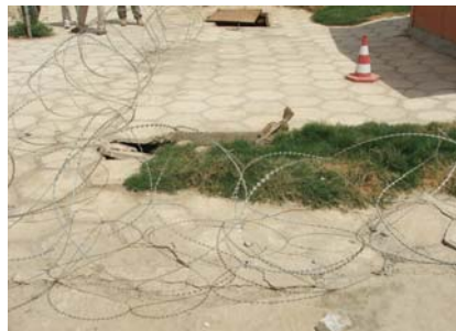
A collapsing septic system at Hilla Police Academy: an example of poor construction under contracts awarded to Philip Bloom.
