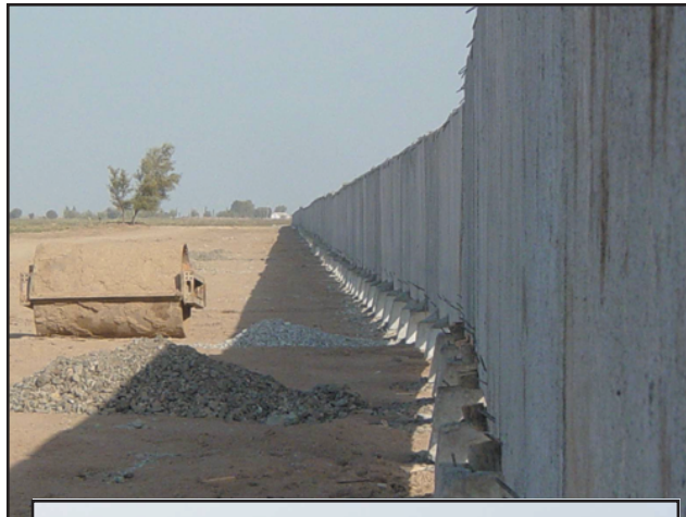
□ Below, this 15-mile-long cement blast wall that surrounds the perimeter of Camp Stronghold Freedom was constructed by a local contractor. In the bottom photo, Afghan workers begin construction of a culvert in Mazar-e Sharif, Afghanistan.
