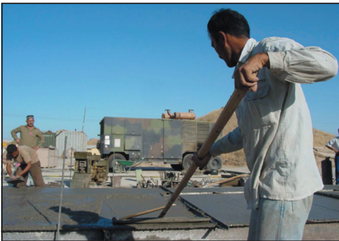
□ At top, local Uzbekistani workers lay cement for power generator platforms. Civilian contractors then will replace the existing Army power-generation unit. Above, one of the workers removes air bubbles from one of the platforms.
