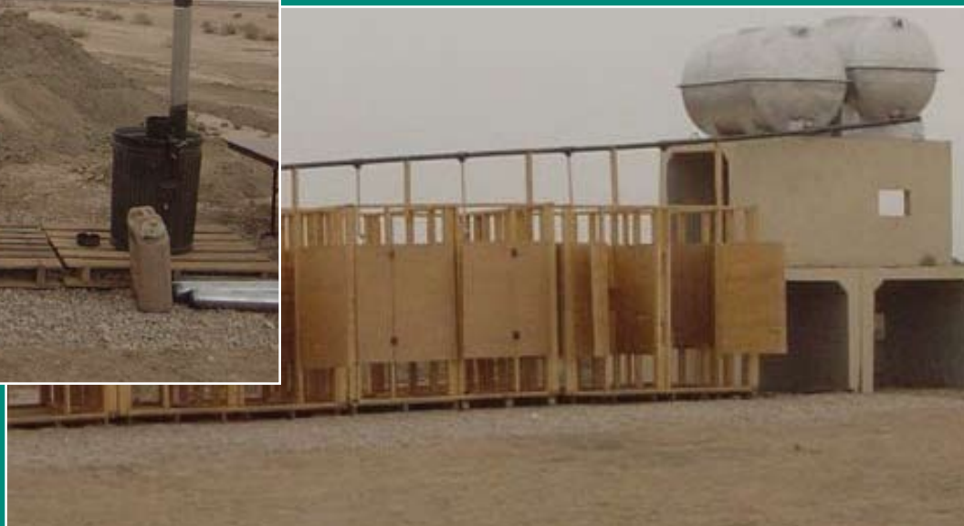
Immersion heaters (above) provide hot water for food preparation and showers (at right) in the field.
