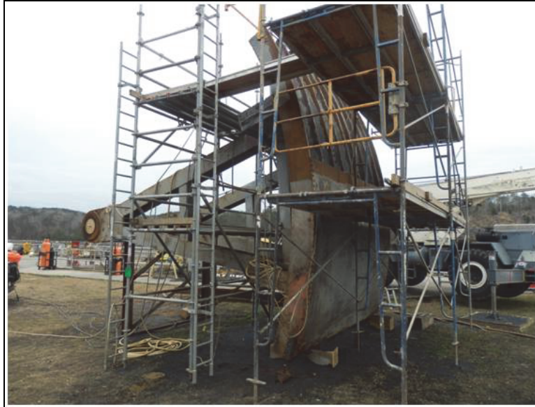
Figure 3. Replacing upper skin plate on Bankhead Lock valve.
