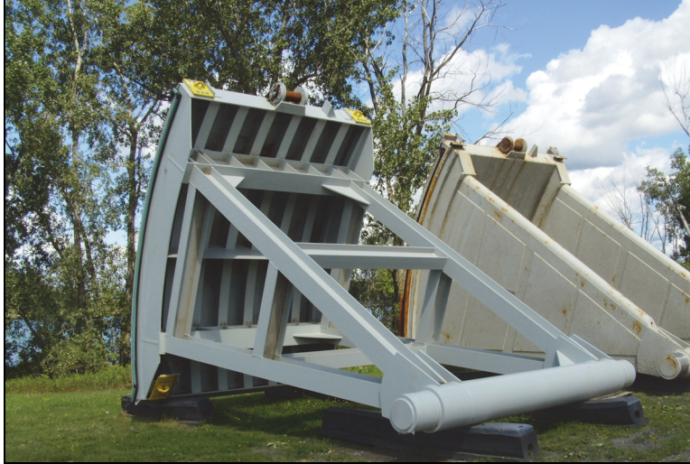
Figure 1. Valves on the Eisenhower and Snell Locks: new vertically framed design in foreground, existing double-skin-plate design in background.
