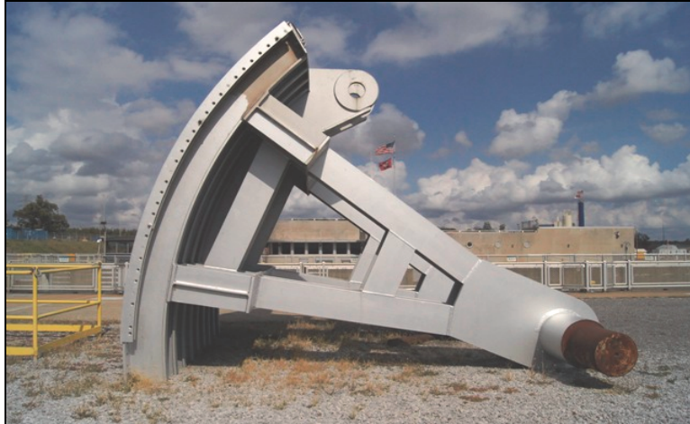
Figure 5. Kentucky Lock replacement valves.
