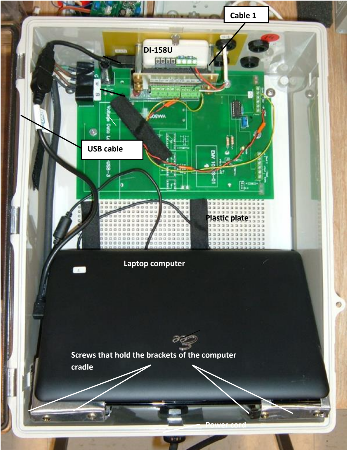
Figure 3. Readout/power module with cables connected.
