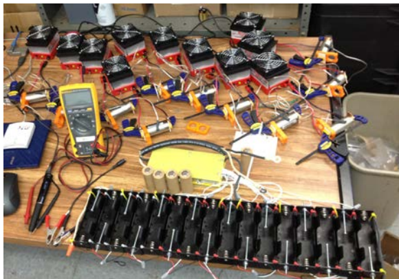
Figure 8: CBA units and rapid-deployment battery module
