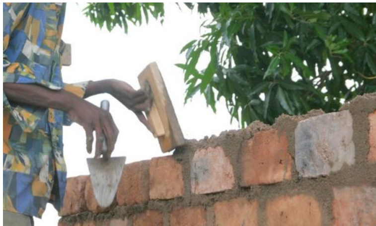
Figure 13. Traditional brick and mortar construction (Brice Blondel).
