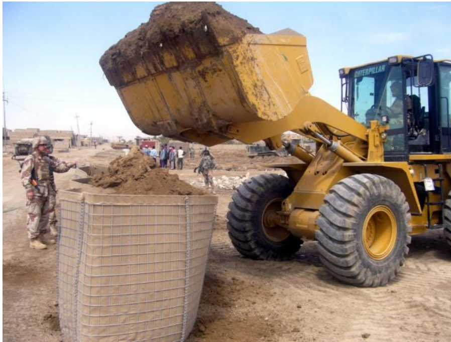
Figure 30. Filling of HESCO bastions in Iraq (US Army).
