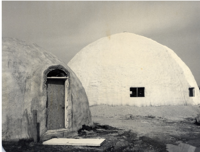
Figure 18. Example of military foam dome application.
