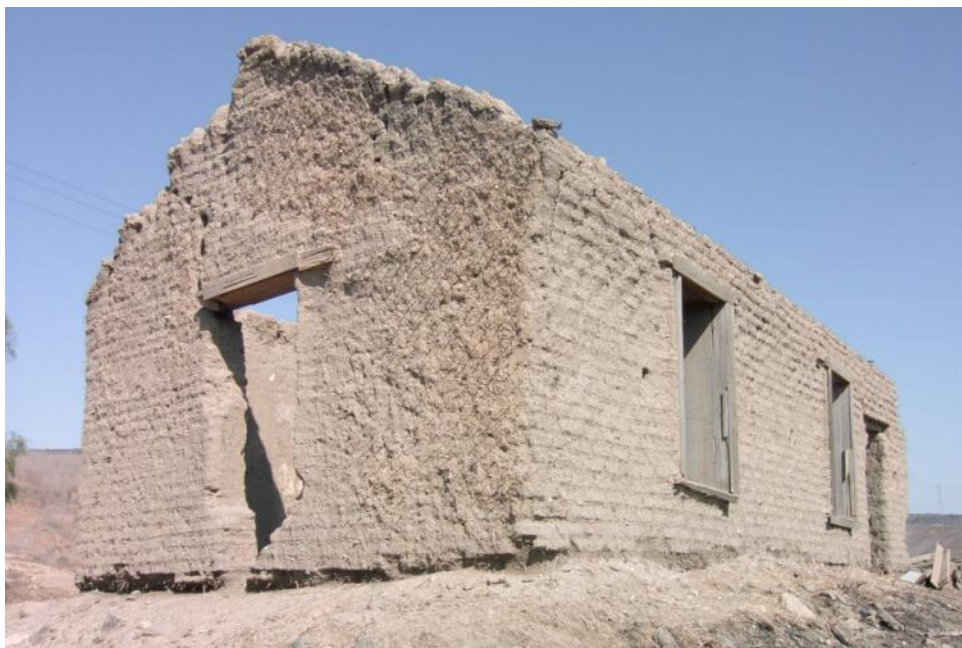
Figure 20. Adobe brick structure.
