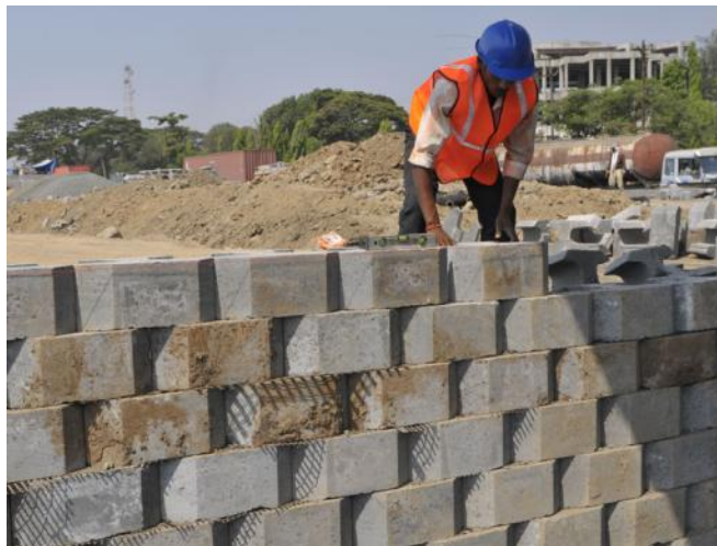
Figure 14. Interlocking mortarless masonry bricks (Dujon Fernandes).
