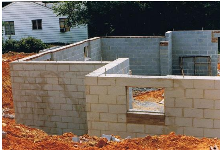
Figure 12. Example of conventional CMU construction.
