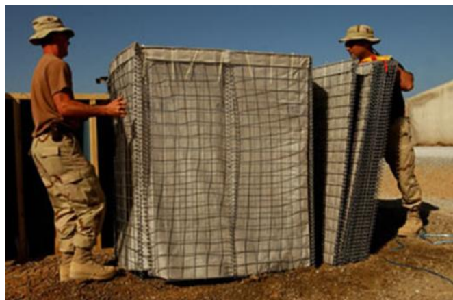
Figure 29. Hesco bastion prior to placement and filling (US Army photo).
