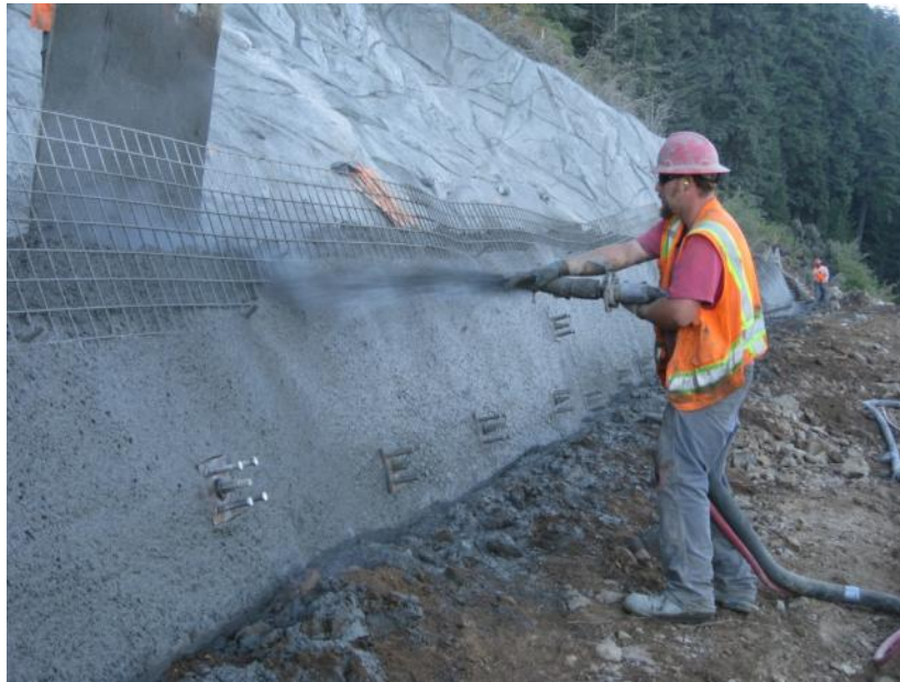
Figure 19. Shotcrete placement (WSDOT).
