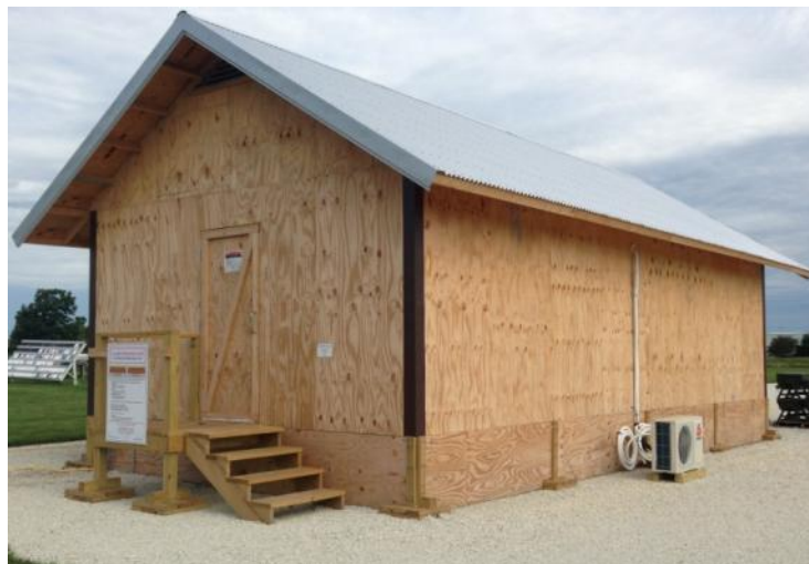
Figure 11. Typical wood-frame B-Hut.
