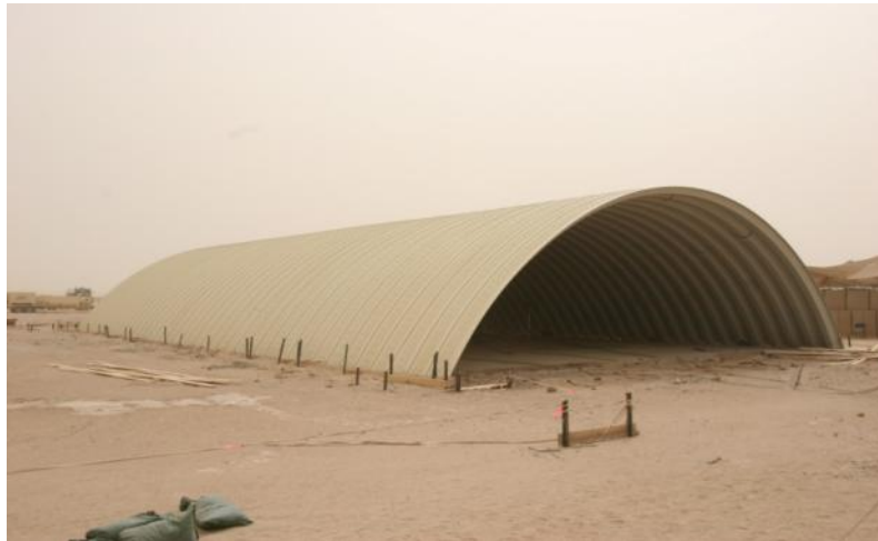
Figure 15. Typical military K-span structure (US Marines).
