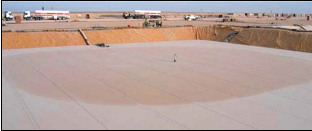
Figure 1. Typical coated fabric fuel/storage tank, showing wet spot on top panel surrounding the pressure release valve.
