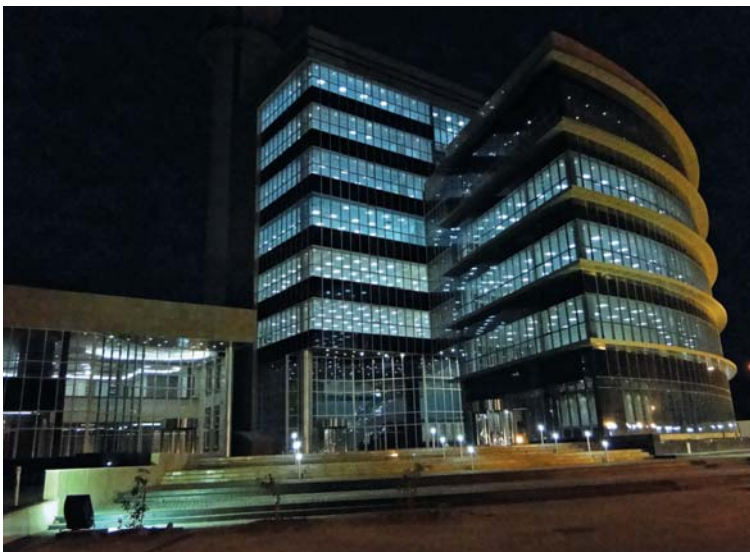
The $18.3 million al-Mamoon Exchange and Communications Center in Baghdad was turned over to the GOI on June 30, 2011, almost five years after its originally forecasted completion date. (USACE photo)
