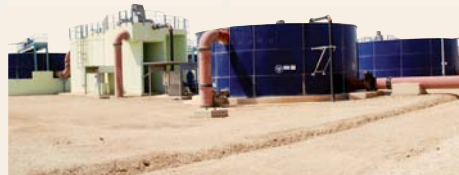
After: Completed WWTP in 2011
