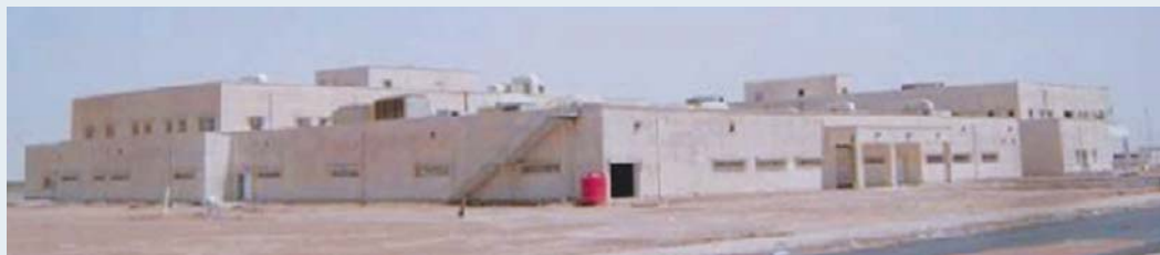
USACE expected to complete ESF-funded construction of the Missan Surgical Hospital by the end of 2012. (USACE photo)
