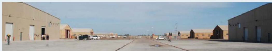
The Depot Distribution Central Operation storage facilities at Camp Taji was completed in November 2010. (USACE photo)
