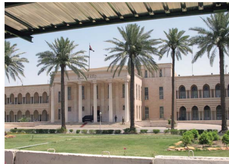
The renovated Iraqi Ministry of Defense headquarters in Baghdad.
