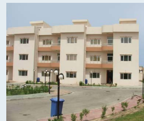
The quality of work at the U.S.-funded project in Erbil was the best SIGIR ever observed.
