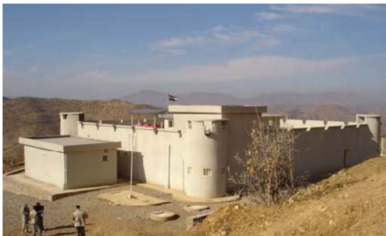
SIGIR conducted project surveys of 21 border forts located along the Iraq-Iran border.
