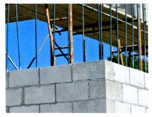
The same wall as above showing double rebar at the wall's corner. *RE photo*.
