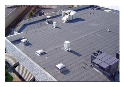
Figure 11. Typical "flat" roof with air conditioning and ventilation units. Note tar paper strips, parapet, and slight slope to gable roof.
