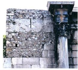
The rubble stone wall, on the left, was covered with thin sheets of stone to give the appearance of ashlar stone. Wall is in Greece. RE photo.
