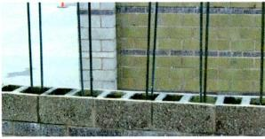
Another method of reinforcement uses two rebars placed in alternate cavities.
