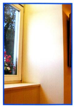
Wall thickness at Ground Floor: 96 cm (8 bricks)
