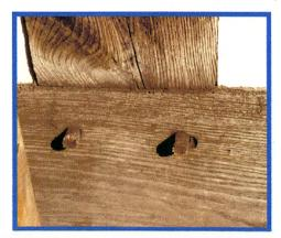
Dowels fix tenon to mortise in this example in the UK. *RE photo.*
