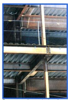
Beam connections and column/beam connections. *RE photo*
