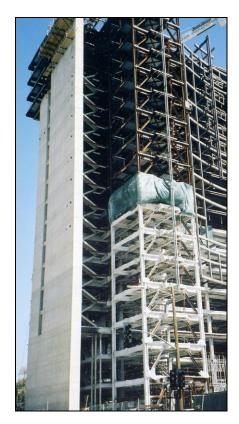
Figure 3. The reinforced concrete end wall of a steel-framed high-rise office building.
