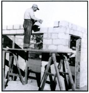
Top row CMUs being laid in construction of a single story building. No rebar has been used in its construction. This form of construction is common for single story structures in Third World countries.
