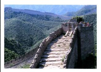
China's Great Wall manifests the principle that a wall exterior will employ ashlar (dressed) stone while rubble stone is used in the interior. The roadway on the wall top, on the right, has disintegrated to the point where vegetation is growing in the exposed soil. Note the use of brick for the castellated walls. RE photo
