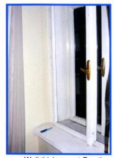
Wall thickness at Fourth Floor: 48 cm (4 bricks)
