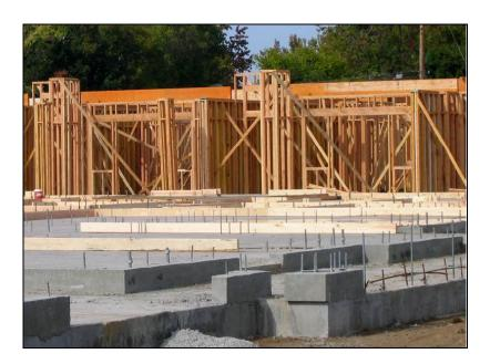
Figure 5. Wood-framed structure being built upon a reinforced concrete base. This is the same structure as in figure 4, at a more advanced state.
