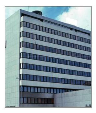
Figure 7. A framed, light-clad office building with a spandrel window pattern. Glass, both clear and opaque, lies between vertical mullions.
