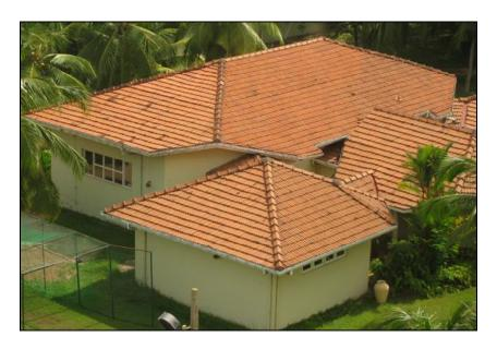
Figure 25. Ribbed terra cotta tile hip-roof on a CMU construction in South Asia.
