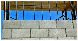
Two cavity CMU blocks have a single rebar in each cavity. Grout has been poured and tamped as each course is added. Maximum construction here meets earthquake code in California. *RE photo*.
