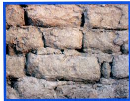
Close-up of Mud Brick Wall Using English Bonding
