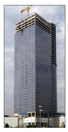
Figure 9. An example of a curtain wall being placed on a R/C-framed office building. Glass, clear and opaque, is being placed between narrow spandrels and mullions.
