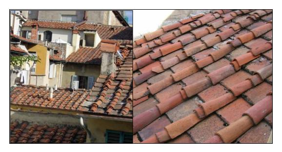
Figure 24. Terra cotta–tiled roof in southern Europe. Detailed photo shows a common practice of convex tile placed over flat tiles.
