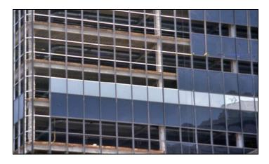
Figure 10. Clear and opaque glass form a curtain wall being installed on a framed office building.
