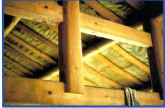
Purlins and truss of the house to the left. The vertical beam is mortised on to the purlin. *RE photo*.
