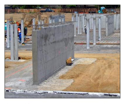
Figure 4. Reinforced concrete shear walls in the basement parking area of a framed building while under construction.
