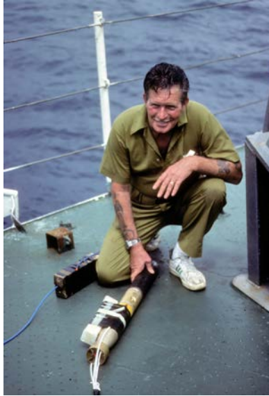
Jason Husty Taylor preparing an impulsive acoustic source line array for reverberation experiments aboard HMNZS Tui in 1979 (Courtesy Dr. B.B. Adams)
