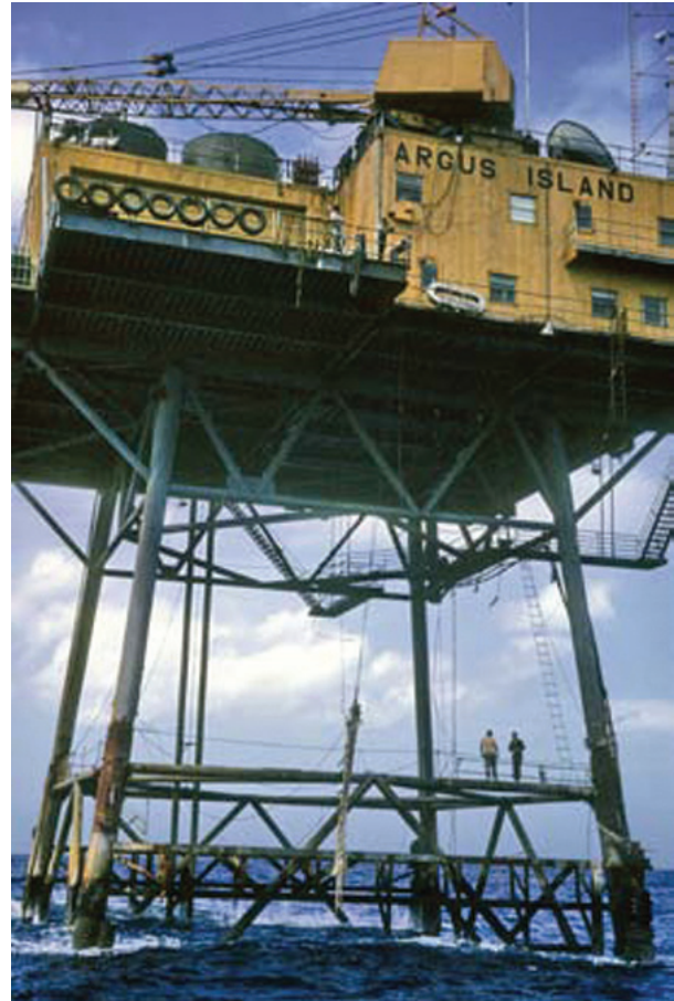
Argus Island tower on Plantagenet Bank near Bermuda where underwater receiver array cables came together for Project Artemis.
