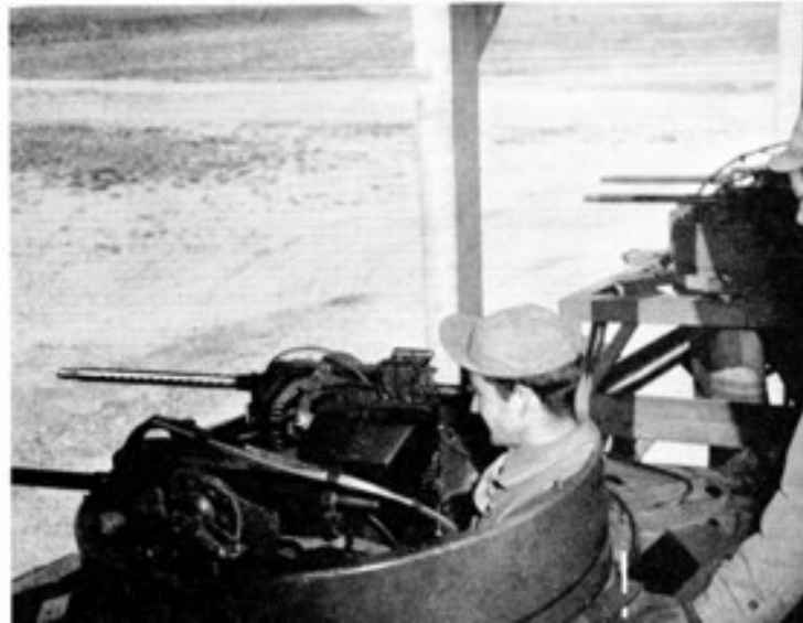
Students, Using Shotguns Specially Mounted on Turrets, Learn How to Operate the Turrets as they Fire at Clay Pigeons Released from 40-foot High Towers Photos provided by: Kingman Army Airfield Historical Society
