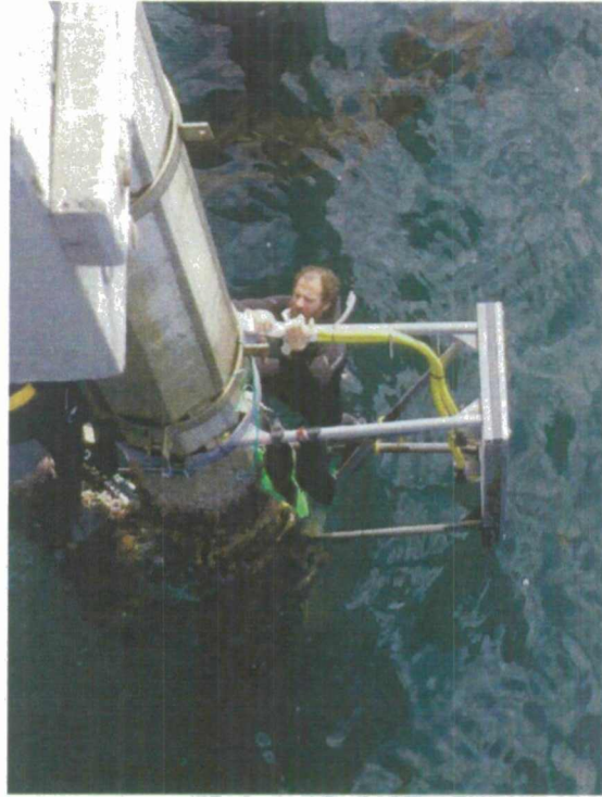
Figure 7. Installation of the plate by divers after being lifted into place by crane.
