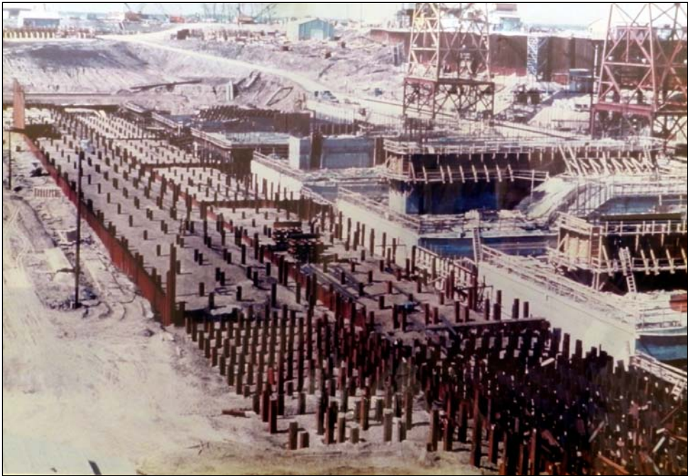
Figure 1.3. Pile layout for spillway at Melvin Price Lock and Dam in St. Louis, Missouri.
