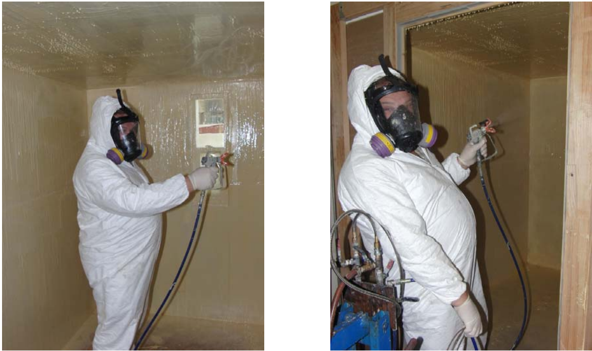
Fig. 10. Testing Shed in the Process of Coating Application
