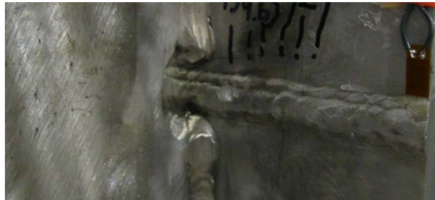
Figure 2. The front of the specimen shows the butt weld and rathole where crack initiation occurs.
