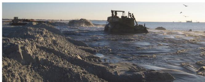
Figure 2. Berm construction: Sand is pumped onto the beach and graded (photo taken December 18, 2011).
