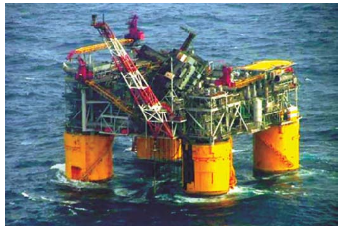
Figure 20. Damaged offshore platform after Hurricane Katrina
