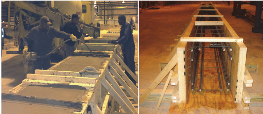
Figure 2. Full scale 4-rod test bed during construction and concrete placement.
