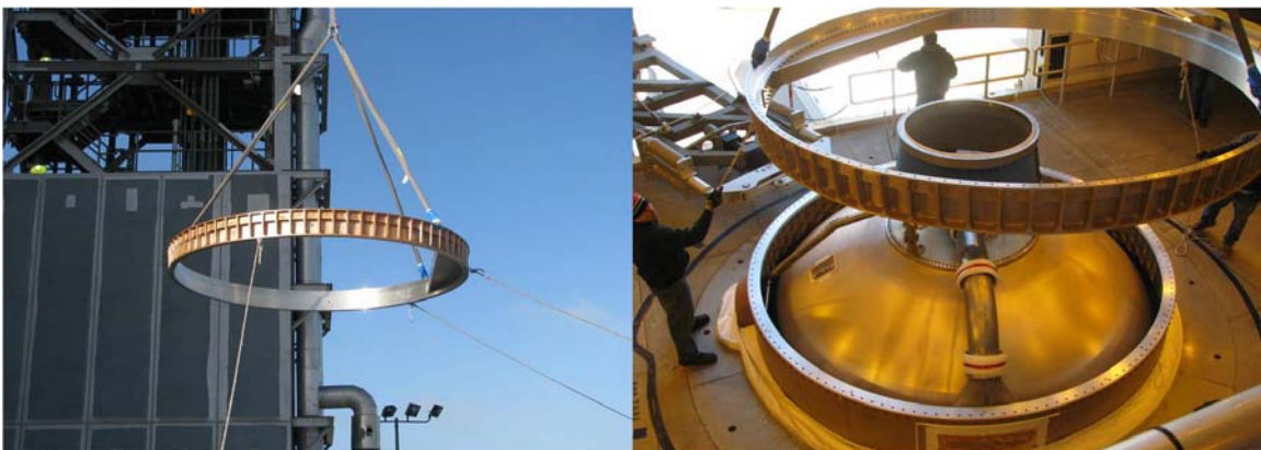
Figure 26. Booster Interstage Adapter Mate
