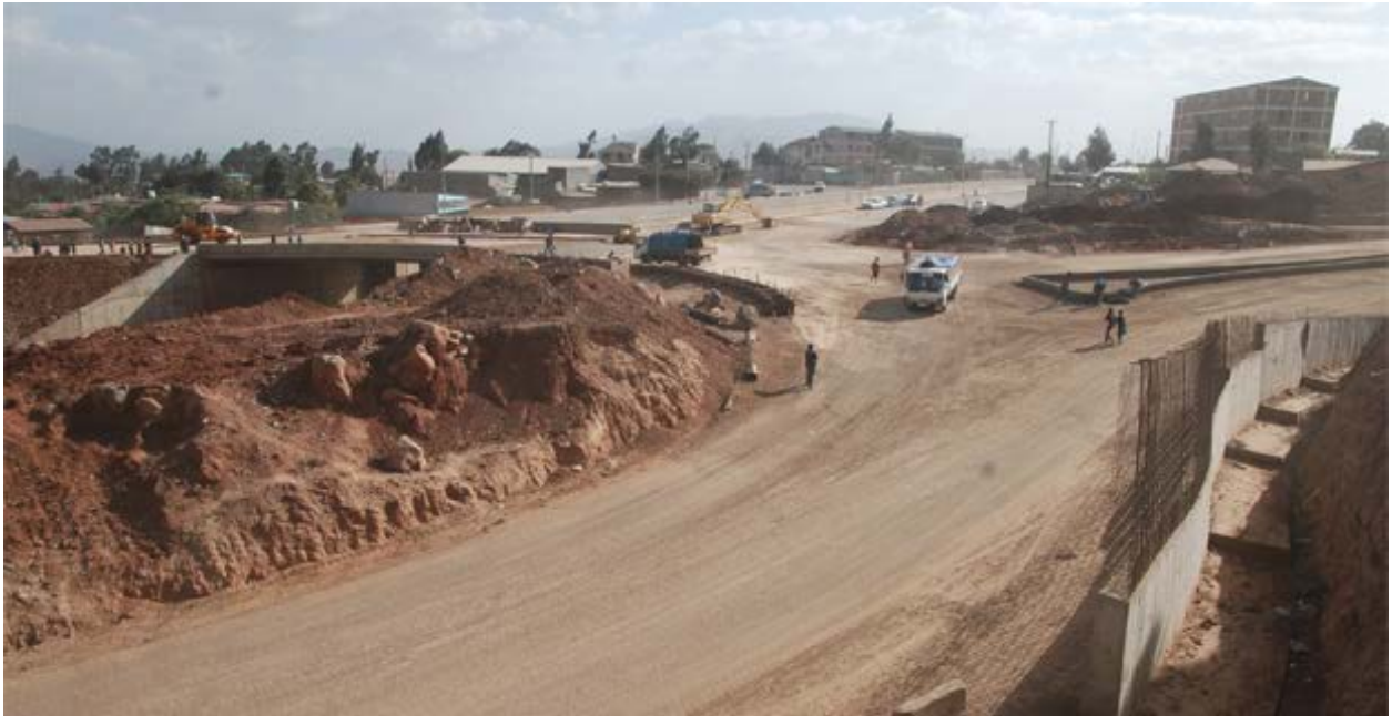
Road Construction in Addis Ababa
