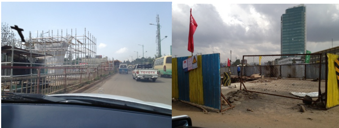
Light Rail Construction in Addis Ababa
