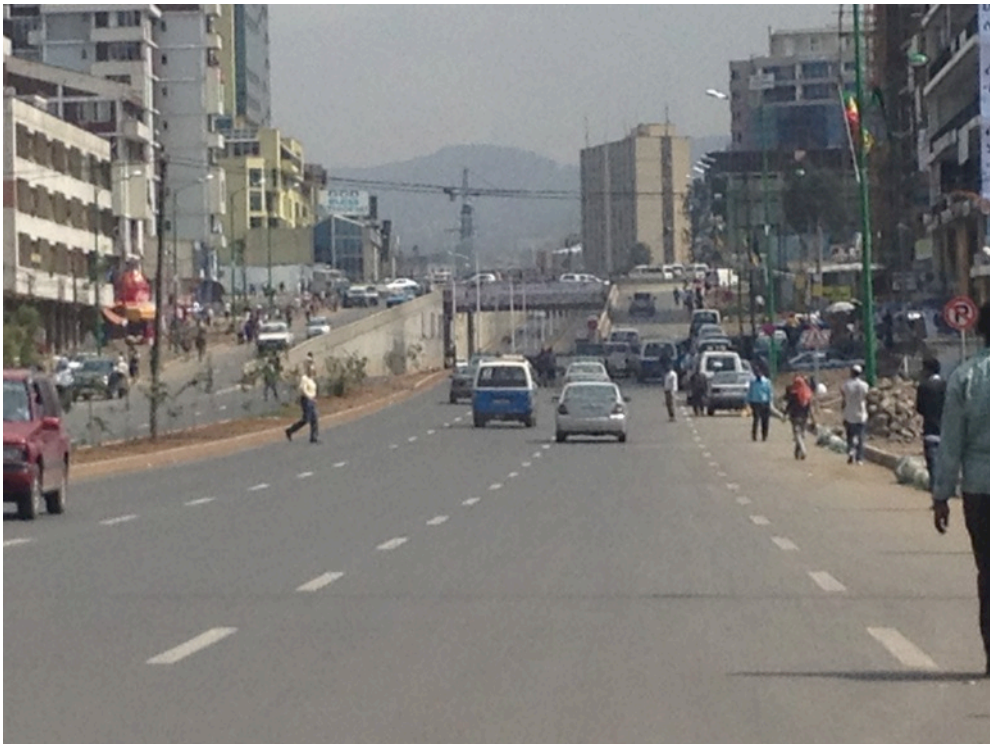
Recently completed Express and Local Lanes Bole Road/Africa Avenue in Addis Ababa
