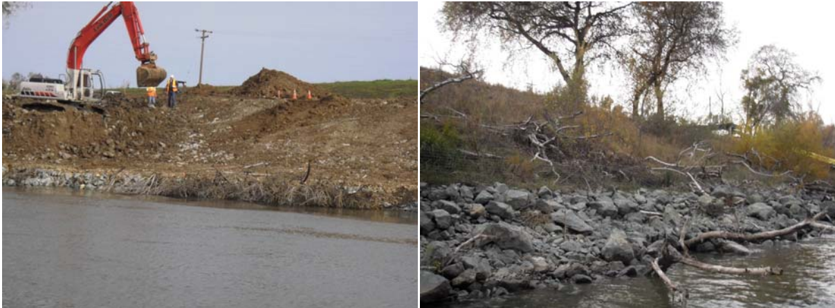
Figure 1. Levee repair site during the restoration (left) and post restoration (right).
