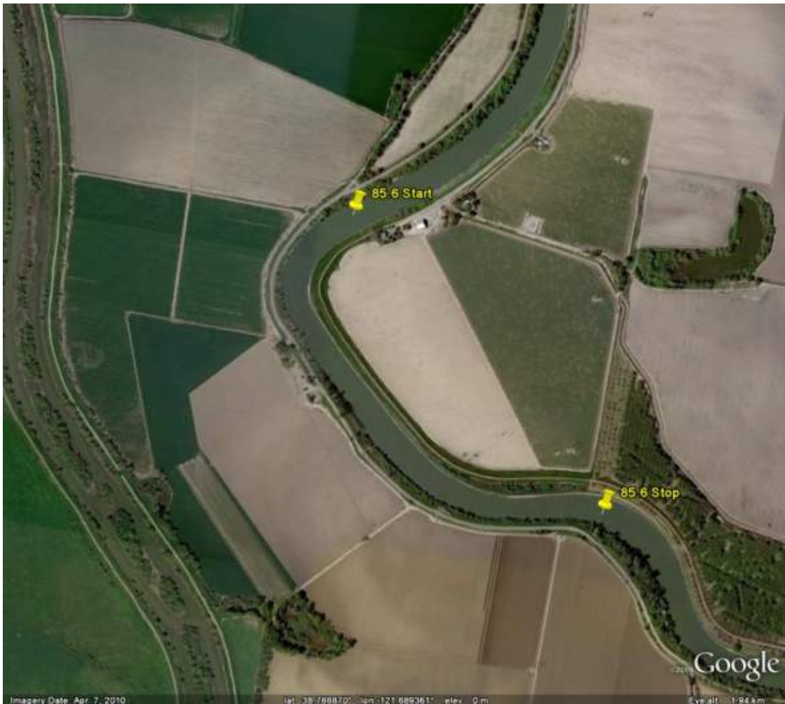
Figure A8. RM 85.6 study area. The levee repair is on the left side of the image (riverright). The levee repair type is a slope with embedded woody material.
