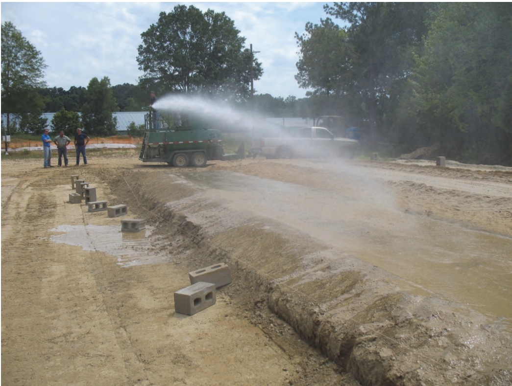
Figure 21. Wetting surface of lift 3 of test item 3 (ML-3) using hydroseeder.
