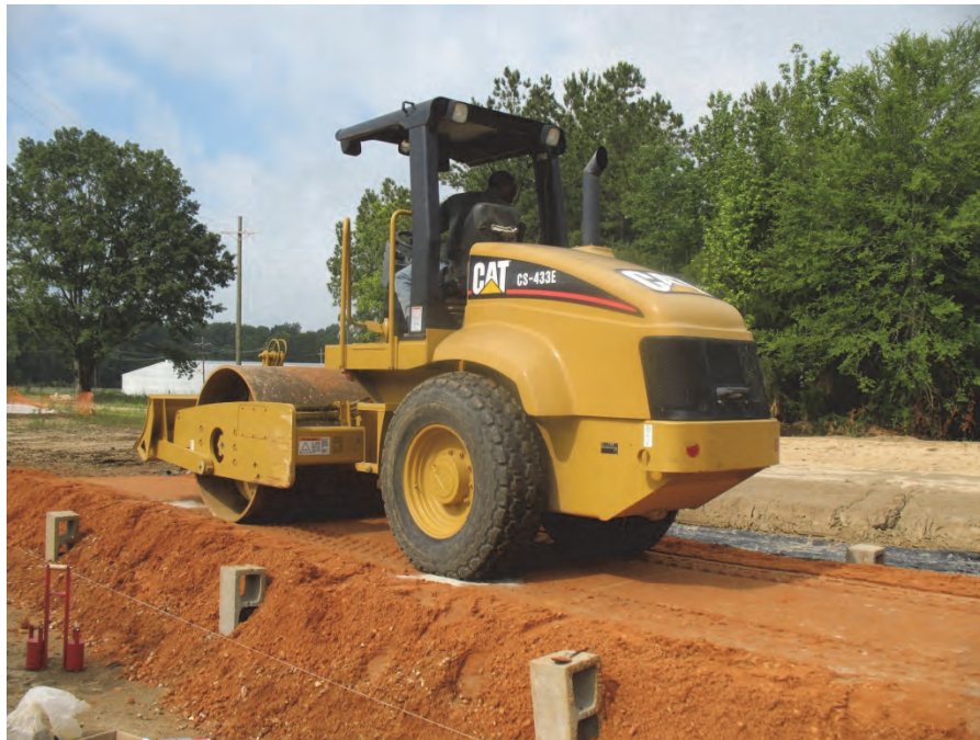
Figure 19. Caterpillar CS-443E vibratory roller used in soil compaction on SP-SM soil. Note string line and cinder blocks to provide thickness control.
