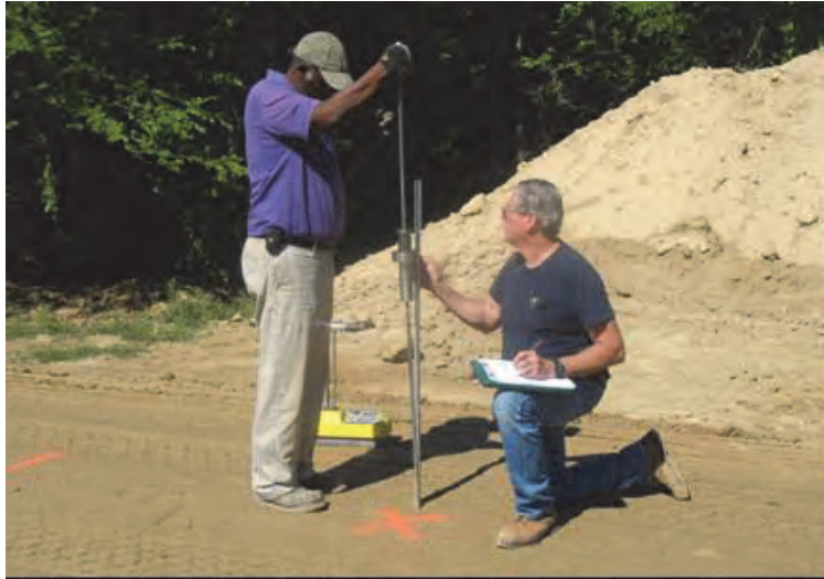
Figure 10. Dynamic Cone Penetrometer (single and dual mass used).
