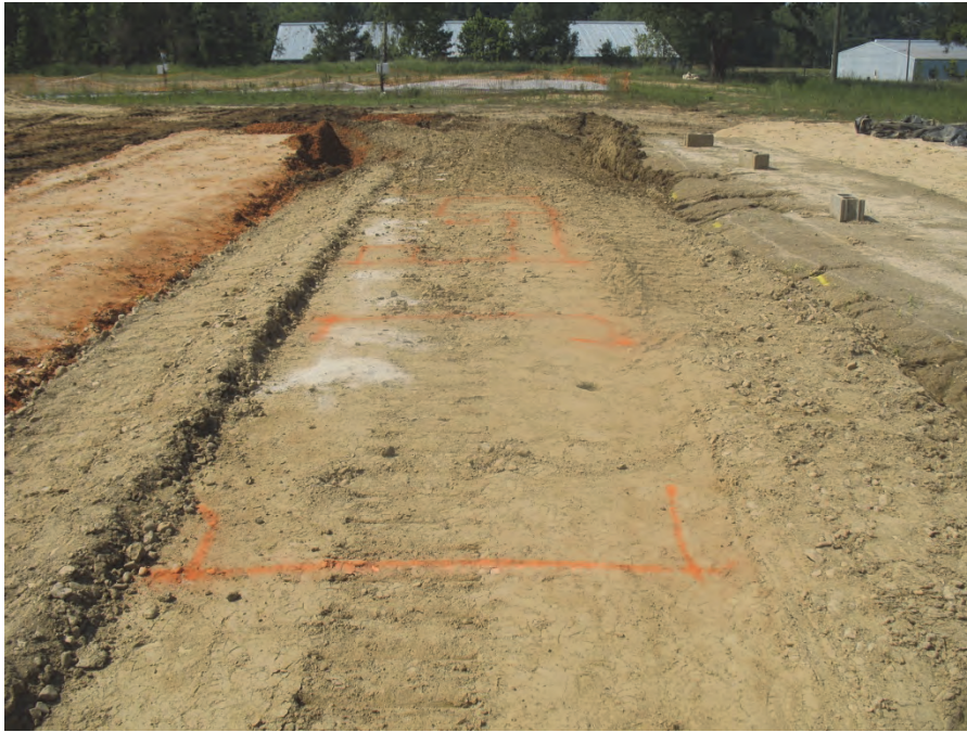
Figure 22. Damage on test item 4, lots 3 and 4.
