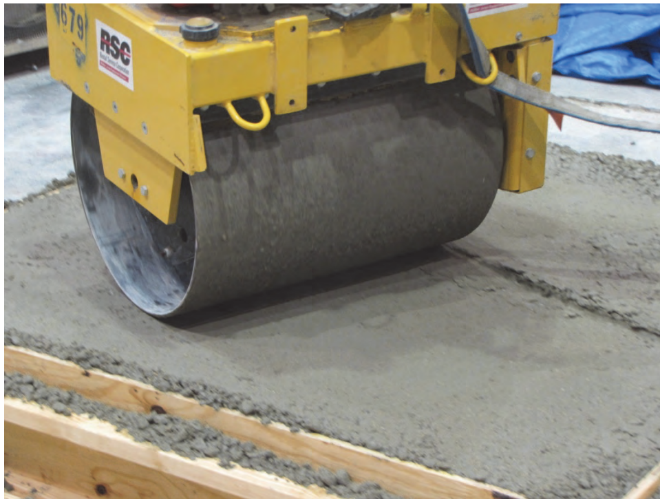
Figure B7. Close image of roller applying smooth surface.
