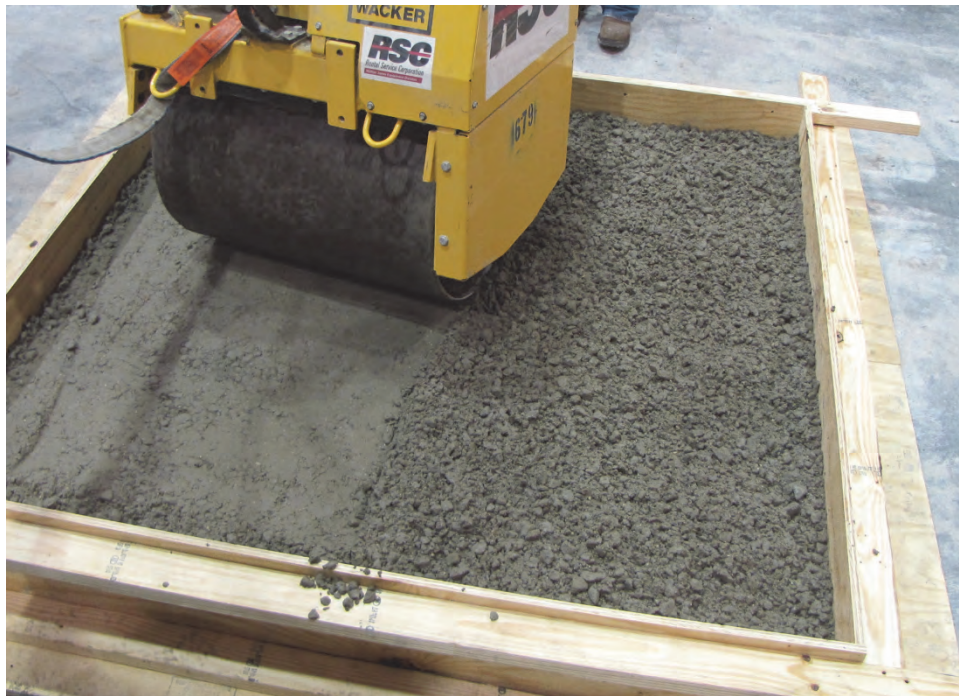
Figure B3. First lift of concrete being roller compacted.
