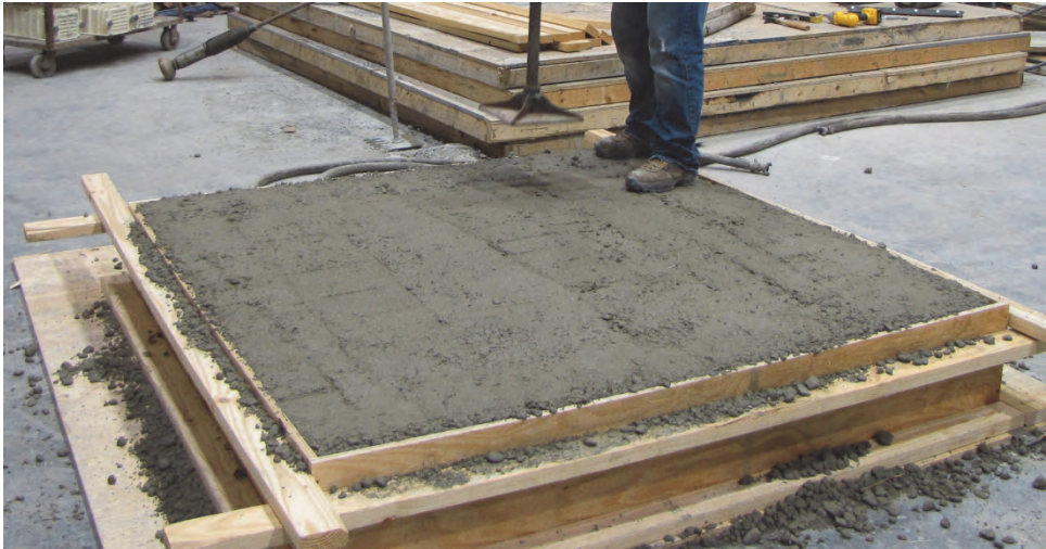
Figure B9. Final surface finish being applied via hand tamps.
