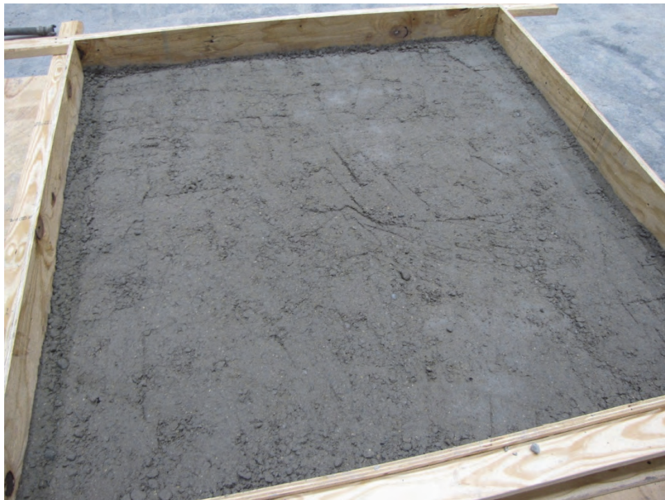
Figure B4. Finished surface of first RCC lift.
