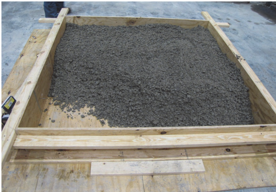
Figure B2. First lift of concrete in forms prior to leveling and compaction.
