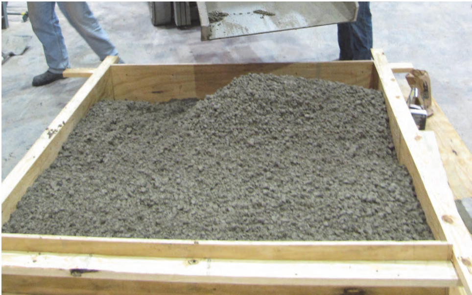
Figure B5. Second lift of concrete in forms prior to leveling and compaction.
