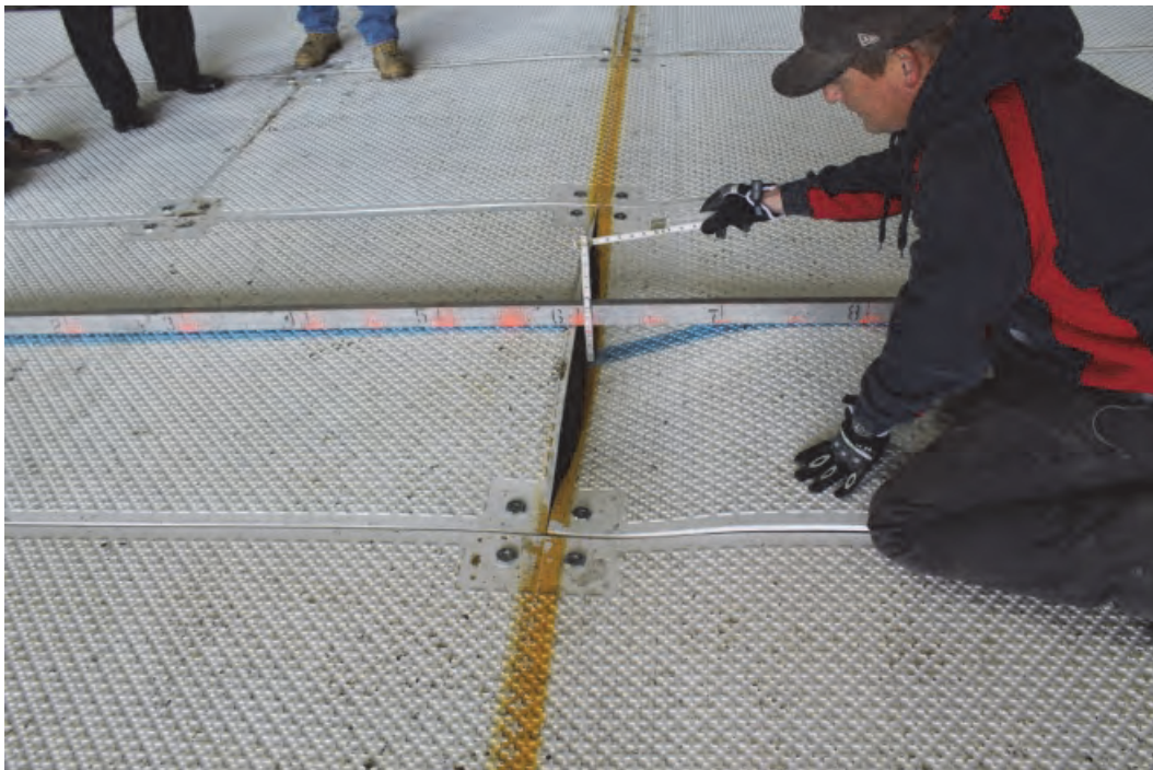
Figure 22. DuraDeck® subgrade deformation after 2 passes on F-15E Lane 1.
