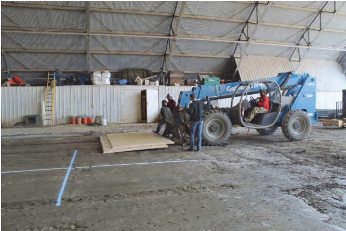
Figure 12. Positioning MegaDeck™ panel with an all-terrain forklift.
