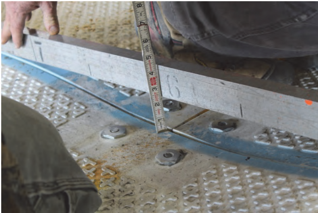
Figure 26. DuraDeck® final deformation on 25 kip forklift lane at connector plate location.
