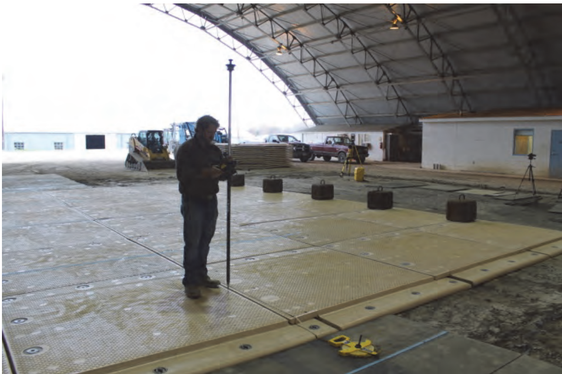
Figure 20. Measuring permanent deformation with robotic total station.
