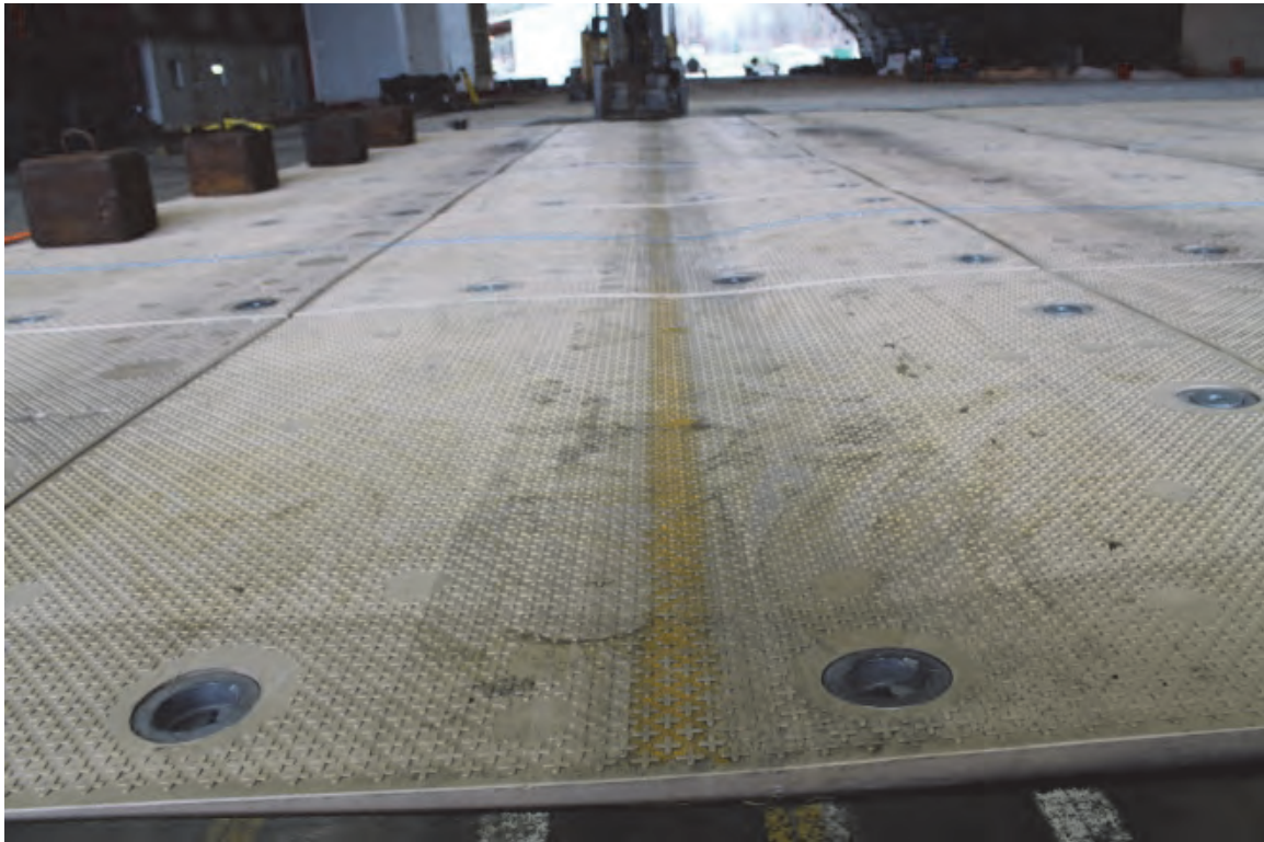
Figure 35. MegaDeck™ F-15E Lane 2 after trafficking was concluded.
