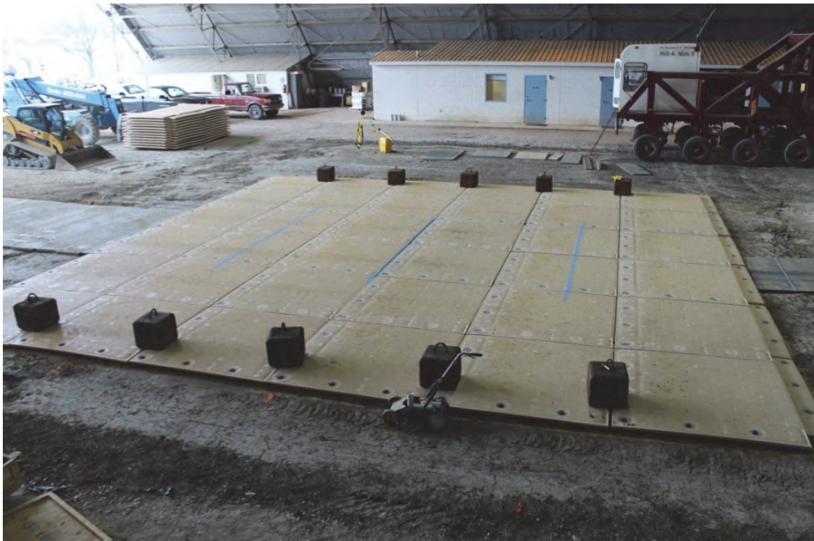
Figure 16. Final layout of MegaDeck™ test section.
