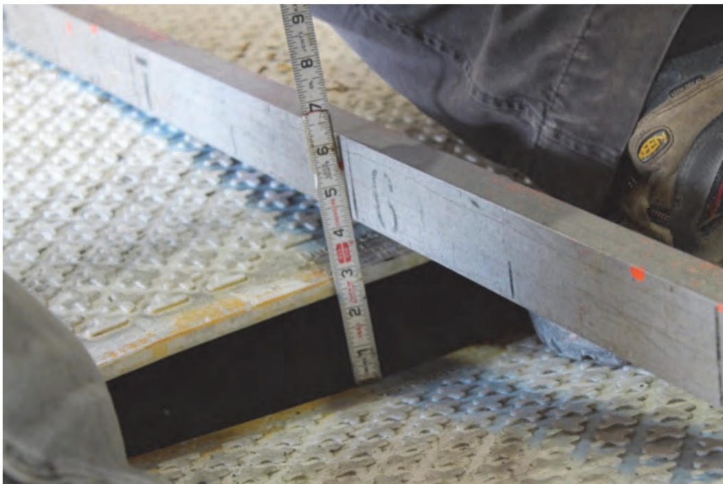
Figure 27. DuraDeck® final deformation on 25 kip forklift lane along unsupported joint.
