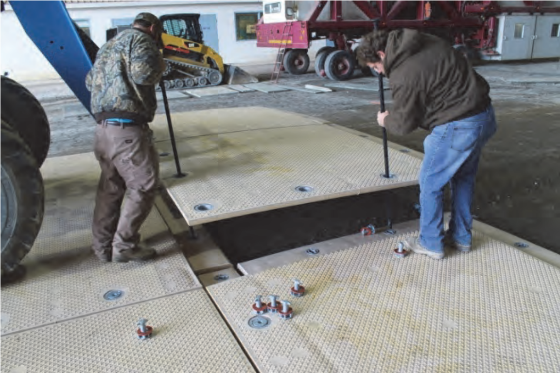
Figure 13. Guiding MegaDeck™ panels into position with guide rods.
