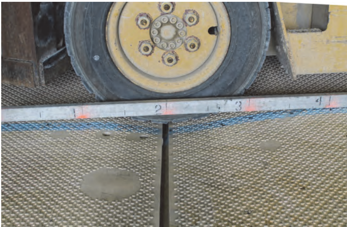
Figure 29. MegaDeck™ final loaded deformation along the joint on F-15E Lane 1.
