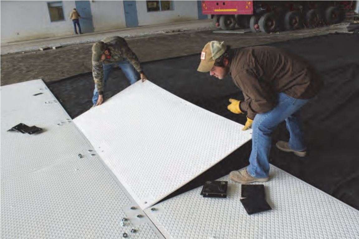
Figure 8. DuraDeck® panel installation.
