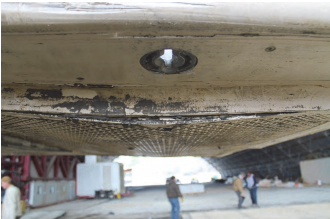
Figure 33. MegaDeck™ bottom skin debonding on F-15E Lane 2.
