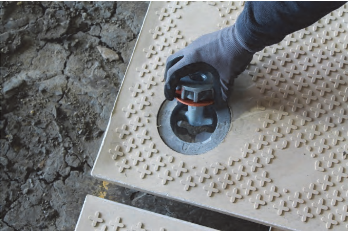
Figure 14. Installing MegaDeck™ connector pin.
