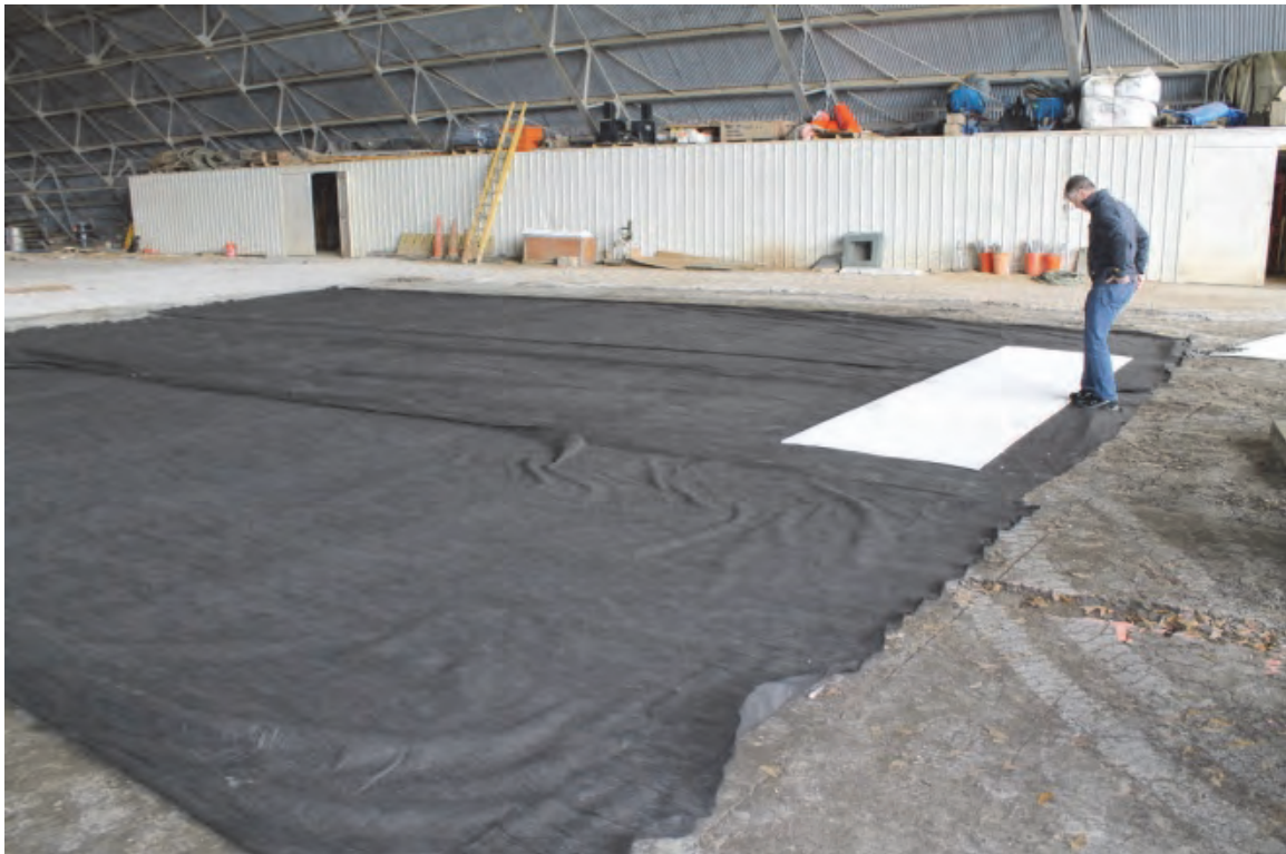
Figure 7. Geotextile-covered test bed.
