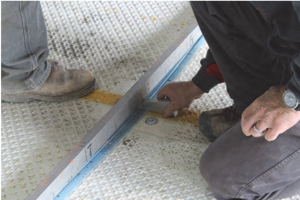
Figure 19. Measuring permanent deformation with straightedge.
