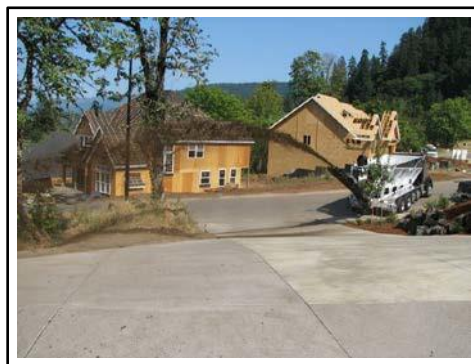
Figure 16. CAS Super Track, direct placement from truck.
