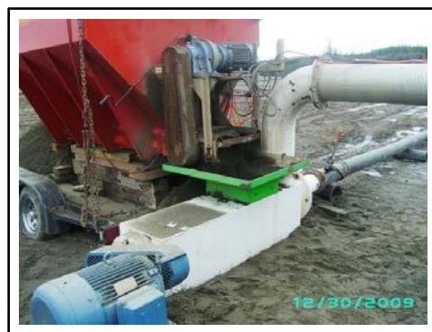
Figure 5. Pneumatic pumping system.
