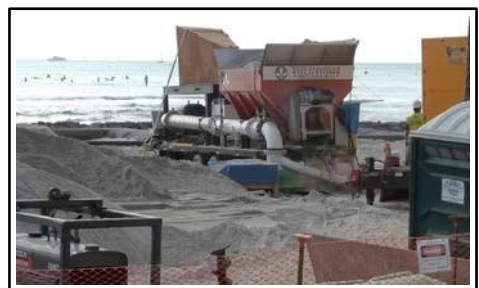
Figure 9. Pneumatic delivery system.
