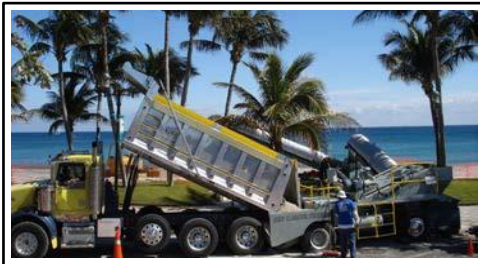
Figure 11. STS dump trucks supplying the feed hopper.
