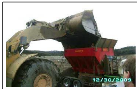
Figure 4. Loading sand into hopper.
