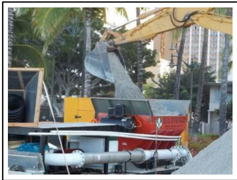
Figure 8. Feeding sand into hopper.
