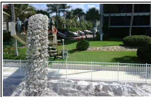
Figure 12. Cascading action of linked conveyor belts.
