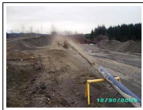
Figure 6. Sand discharging from pipeline.
