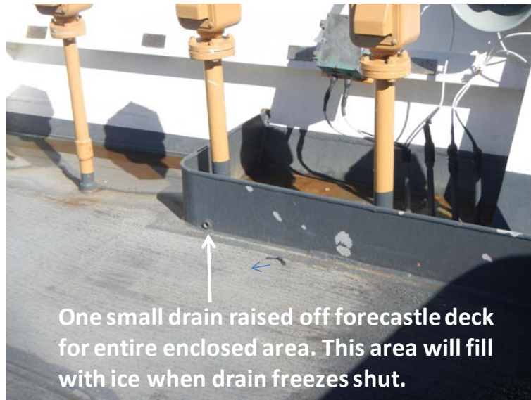
Figure 4-27. Enclosed area at aft end of starboard forecastle with one small drain that can freeze closed (Ryerson 2012).
