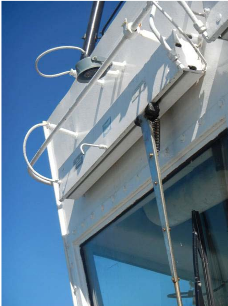
Figure 4-54. Wiper mechanism on bridge windows (Ryerson 2012).
