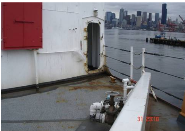
Figure 4-9. Ice accumulates on the forecastle deck ahead of the air castle doors freezing them shut, denying access for anchoring operations (CRREL 2012).
