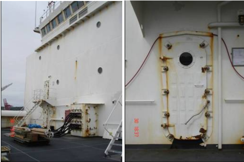
Figure 4-7. High forward bulkhead below bridge cannot be fully de-iced manually (left). Floating ice on forecastle opens watertight doors, allowing water into compartments (right) (CRREL 2012).
