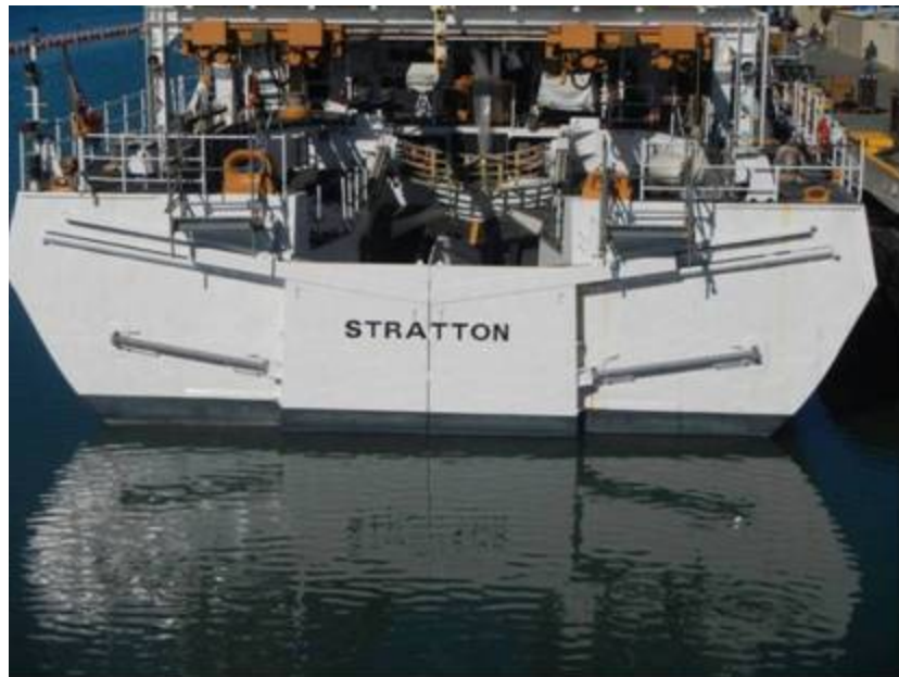
Figure 4-42. Details of BLR System stern doors and vulnerable hydraulic door slides and cylinder mechanism outside transom on NSC STRATTON (Ryerson 2012).
