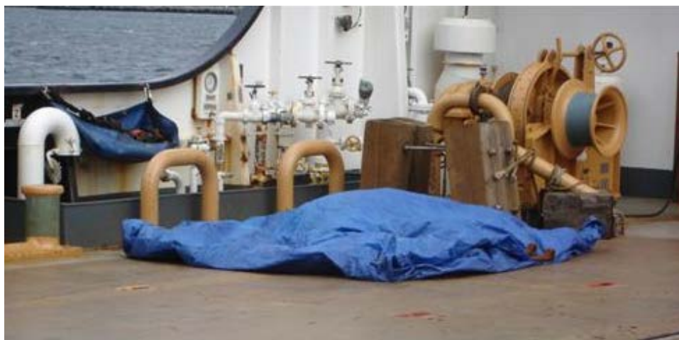
Figure 4-82. Blue tarps used for covering deck machinery (Ryerson 2012).
