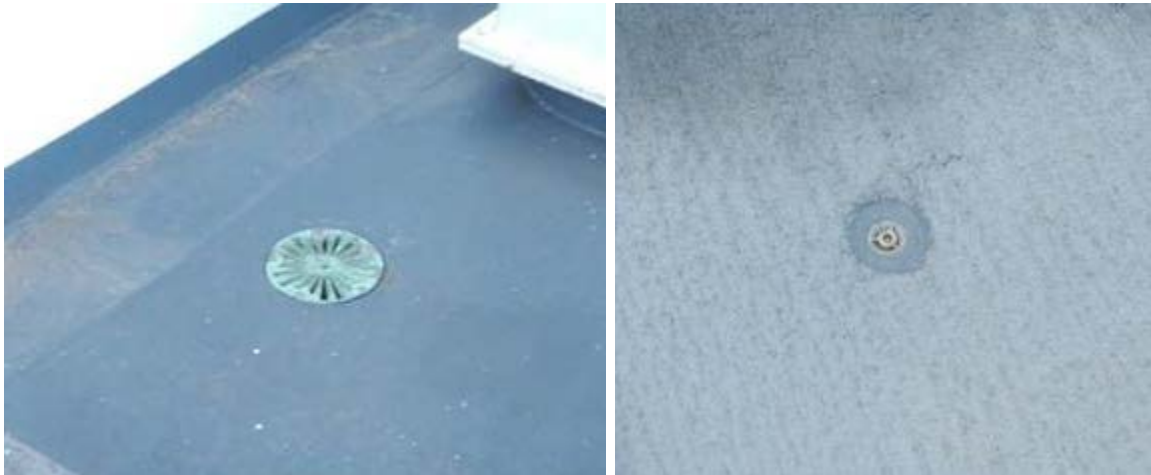
Figure 4.26. Deck drains are often not located in the lowest areas of the deck, they are often clogged with rust and construction debris, and are routed through cold areas that can cause freezing (left). Countermeasure wash-down deck nozzles could freeze, but are not expected to be needed in cold weather (right) (Ryerson 2012).
