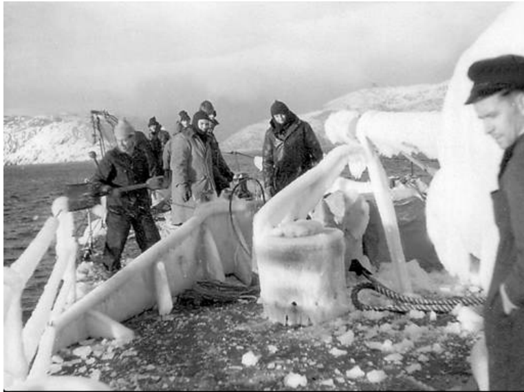
Figure 3-31. De-icing forecastle of HMS Leamington . Photo courtesy of Phil Marley ( www.hazegray.org/navhist/canada/bota/rn/leamington/ ).
