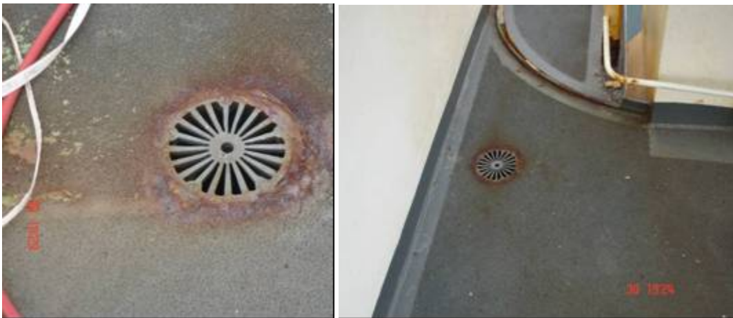
Figure 4-6. Deck drains on the forecastle and in the air castles clog due to rust and ice (CRREL 2012).
