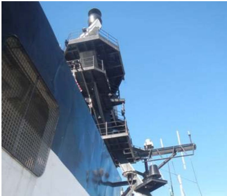
Figure 4-48. Mast with walkways and instrumentation, viewed from Boat Deck on starboard side (Ryerson 2012).
