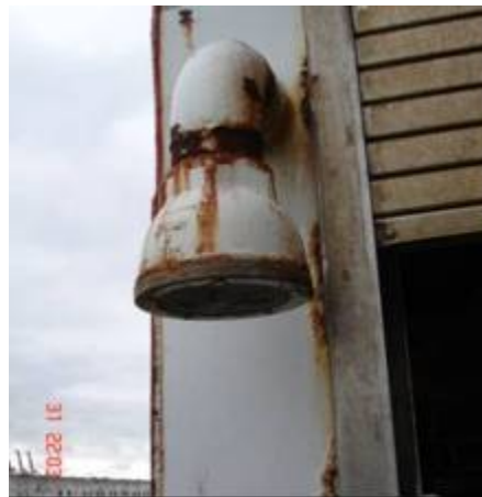
Figure 4-15. Air vents for fuel and water tanks can freeze shut (CRREL 2012).
