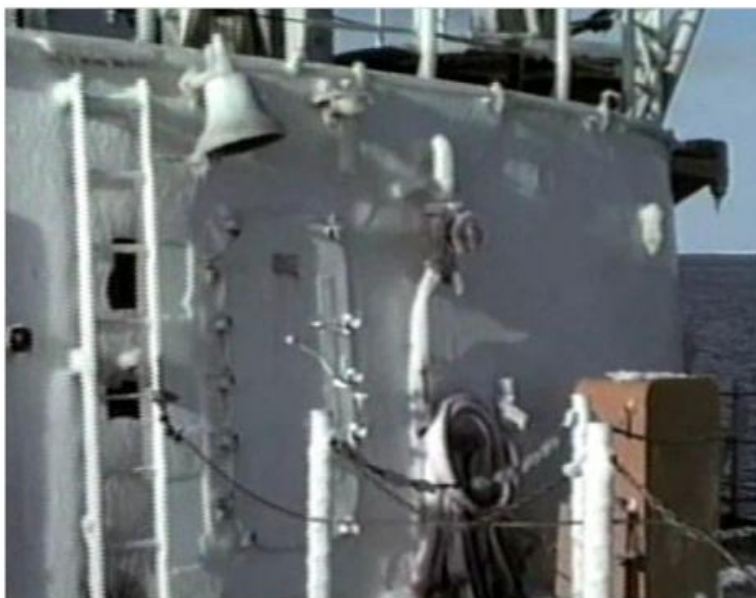
Figure 5-22. Forward bulkhead of CGC MIDGETT after ice had been removed from fire valves and hoses (Ryerson).
