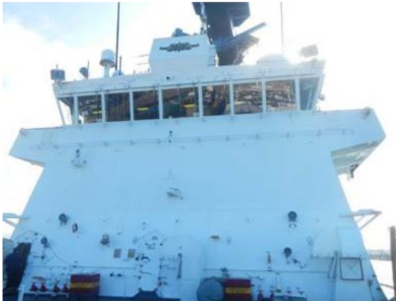
Figure 4-29. Spray reaches bridge in storms. Ice on high forward bulkhead could fall and damage antennas on bulkhead sides, and valves, wires and small piping lower on bulkhead (Ryerson 2012).
