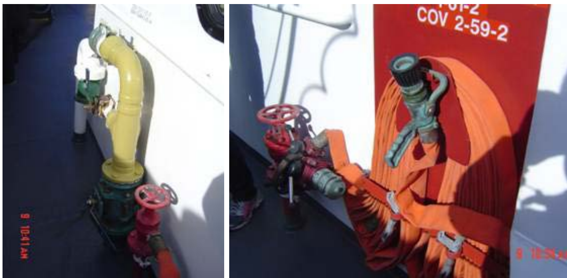
Figure 4-64. Valves and vents become ice covered forward of amidships (left image). Fire hoses are removed before winter because they freeze in place (right image) (CRREL 2012).
