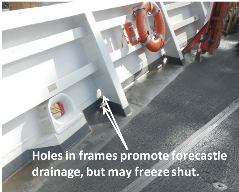
Figure 4-25. Holes in frames promote deck drainage—but may freeze shut (Ryerson 2012).
