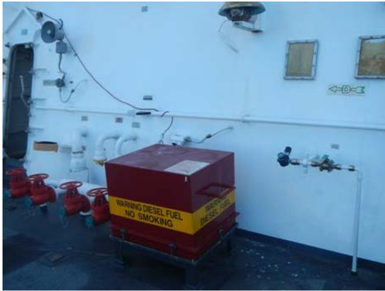
Figure 4-30. Bell and bullhorn cabling, and fire stanchion valves, could be damaged by ice falling from the forward bulkhead (Ryerson 2012).
