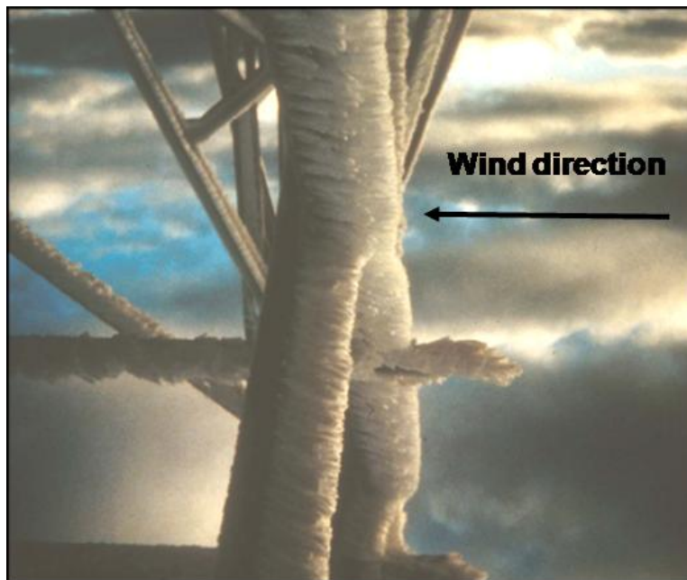
Figure 3-34. Rime ice accumulation on lattice steel structure similar to some components found on ships. Ice on structural shapes is approximately 15-cm thick (Ryerson, n.d.).
