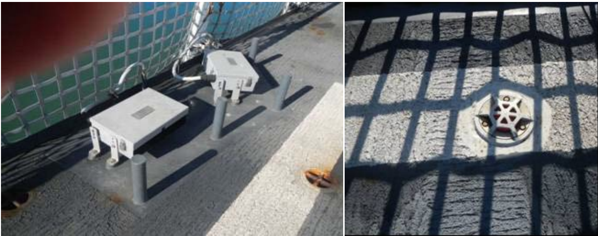
Figure 4-38. Electronic gear and cabling on flight deck could be damaged by snow shoveling. Snow or ice must be removed with care around non-glare landing zone lights for them to be useful (US Coast Guard 2012).
