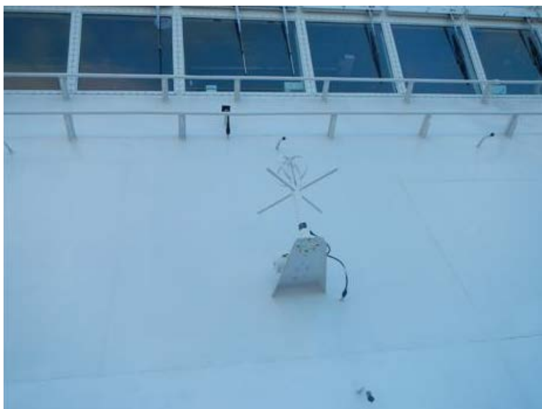
Figure 4-31. Antennas and countermeasure wash-down piping could be damaged by ice falling from the forward bulkhead. Also, antenna performance could be reduced by ice (Ryerson 2012).
