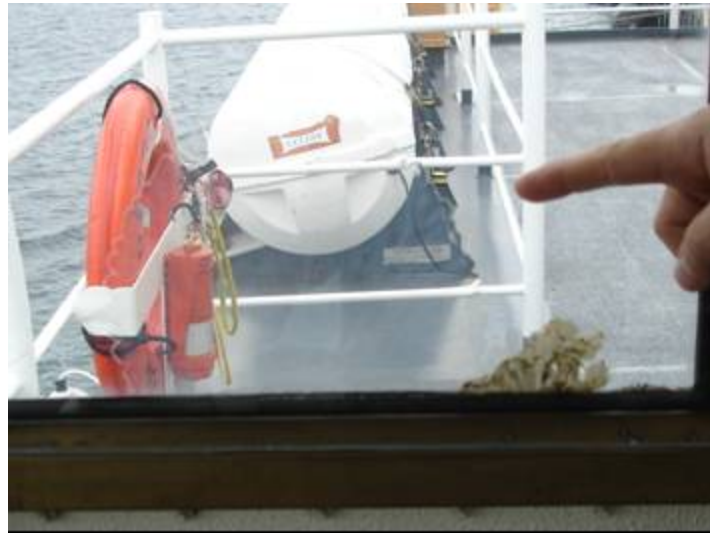
Figure 5-51. Delaminated area of window, opposite fingertip, showing optical distortion, and burned area below finger (Ryerson 2012).
