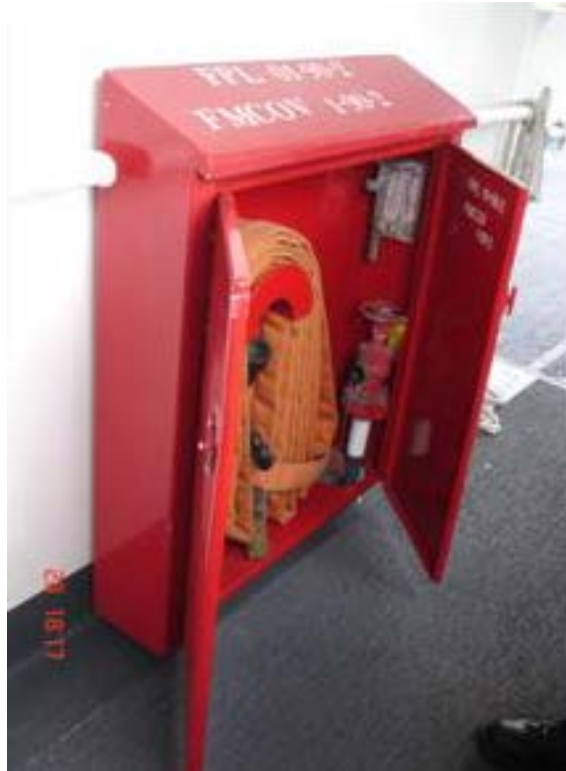
Figure 4-85. Proper metal cover for fire hose and valve on weather deck (Ryerson 2012).
