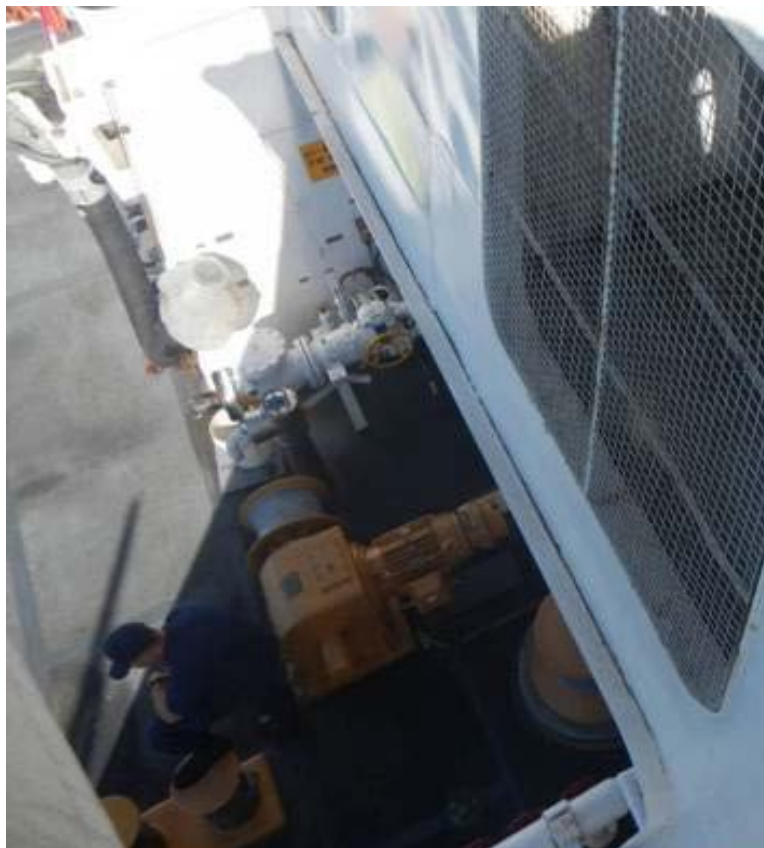
Figure 4-46. FAS deck with piping, winches and hardware that could ice, according to crew, and hinder fueling when underway (US Coast Guard 2012).
