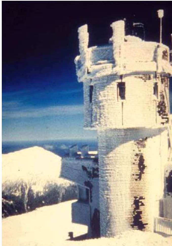
Figure 3-37. Rime formation on tower and whip antennas on Mt. Washington, NH. Note thicker rime ice accumulation on small diameter whip antennas than on large diameter tower structure (CRREL, n.d.).
