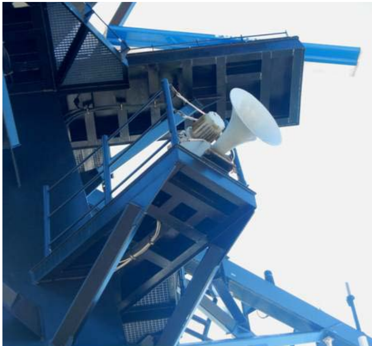
Figure 4-52. Ship's horn with radar above and anemometer on port cross arm (Ryerson 2012).
