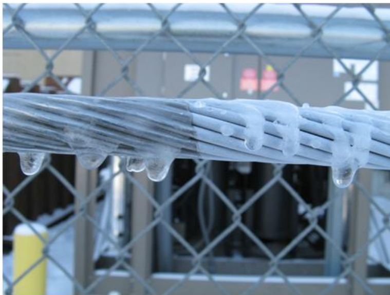
Figure 5-57. Electrical transmission line coated with ISurTec coating right, with bare aluminum surface on left (image courtesy Innovative Surface Technologies, Inc.).
