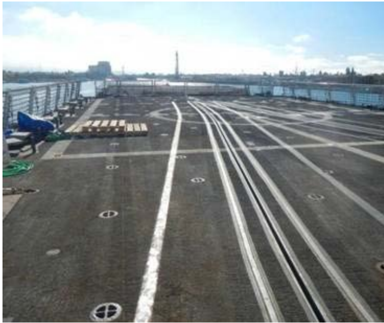
Figure 4-36. Track for guiding helicopters into and out of hangar has not been used, and will be removed. Ice from spray or snow would hinder operation of the system if it were used. Note numerous tie downs in deck that fill with water and could become unusable when frozen (Ryerson 2012).
