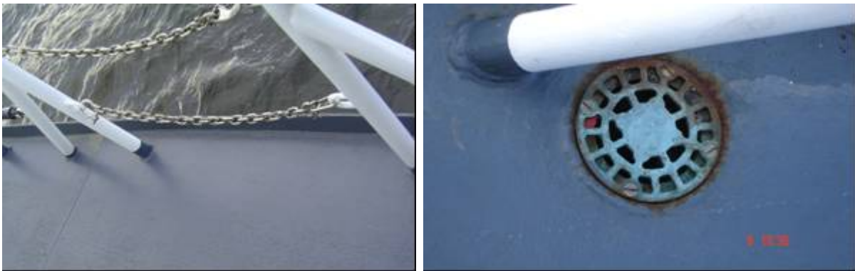
Figure 4-61. Lip along deck edge prevents pollutants spilled on deck from reaching the sea (left image). However, it also reduces deck drainage allowing greater ice accumulation on side weather decks except where there are drains, which never freeze or clog on the THUNDER BAY (right image) (CRREL 2012).
