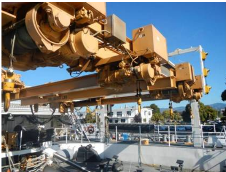
Figure 4-43. BLR system overhead crane (US Coast Guard 2012).
