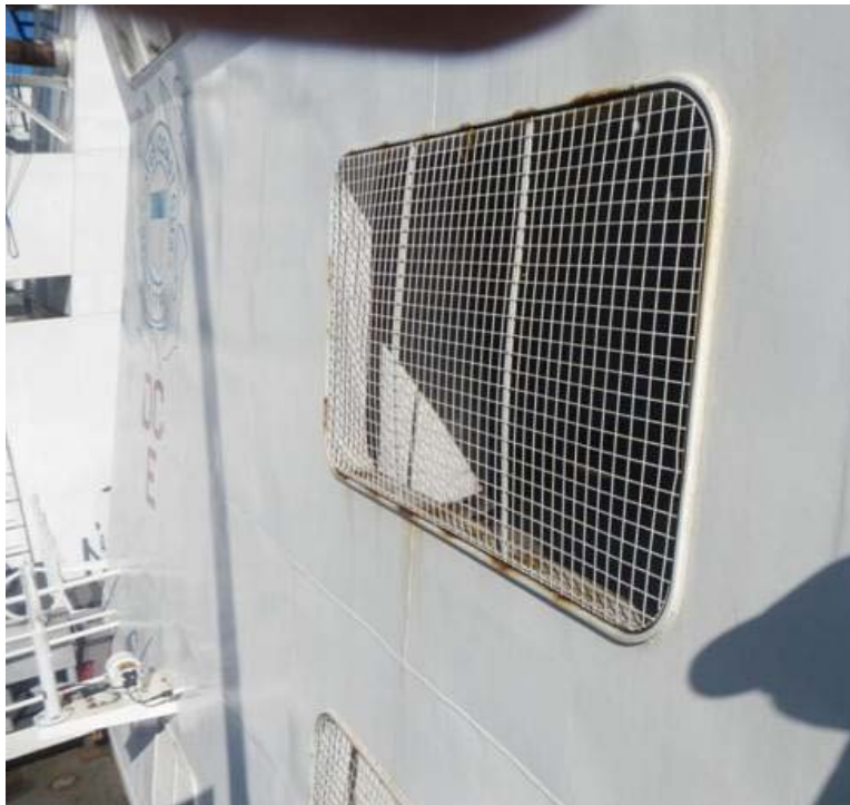
Figure 4-47. Plenum screens above FAS deck on port side. It is assumed that they are exhaust vents because they do not have FOD screens or heating systems (Ryerson 2012).
