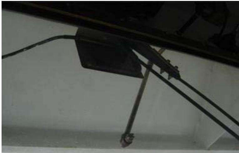
Figure 4-79. Complex window washer/wiper mechanisms freeze and fail on other cutters, but CGC WILLOW has had no problems with them because little icing occurs at the bridge as it is so high and located so far aft (Ryerson 2012).
