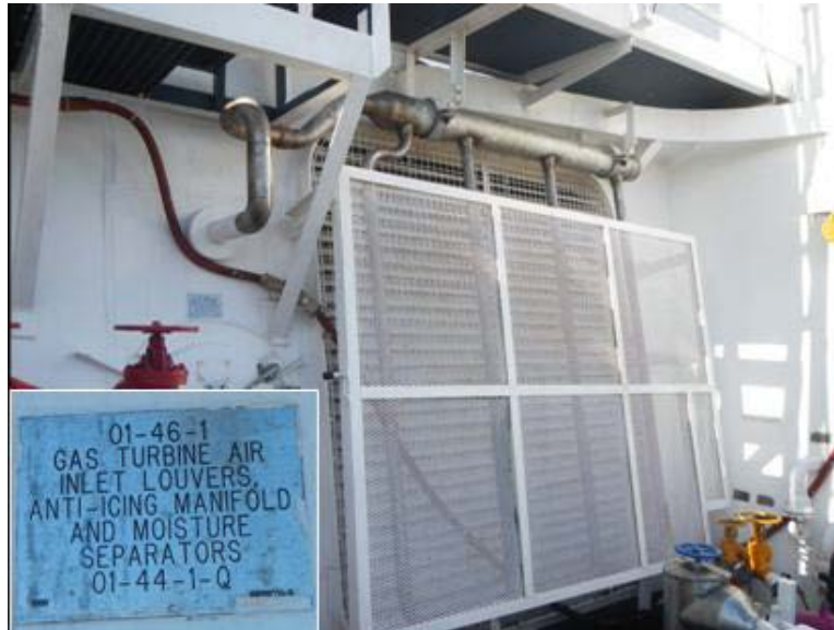
Figure 4-35. Gas turbine air intake on boat deck. A heated manifold behind the FOD screen is intended to keep the intake louvers de-iced. It is not clear how the FOD screen is de-iced (Ryerson 2012).
