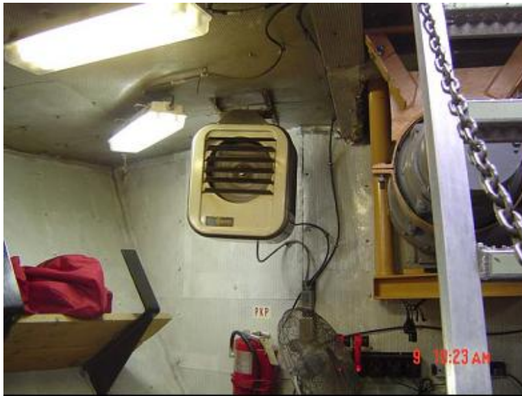
Figure 4-63. Space heater used to heat space under forecastle deck to reduce icing and help de-icing (CRREL 2012).
