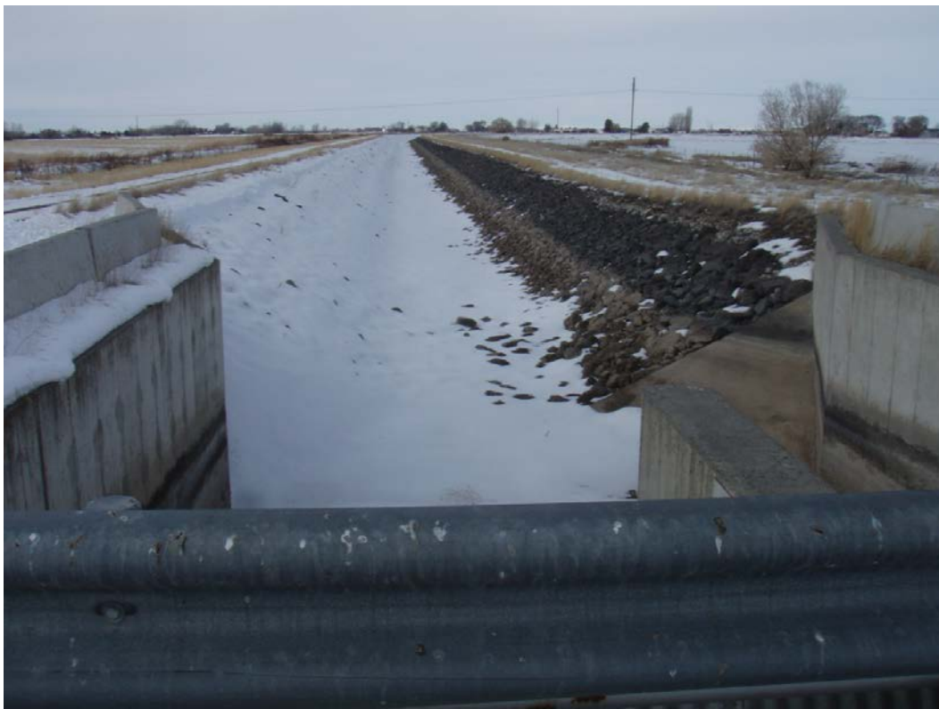
Figure 15. Looking downstream from the Bifurcation Control Structure prior to release. (Image by P. Cooper.)
