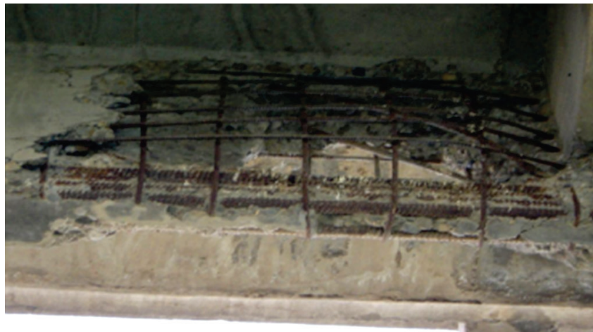
Figure 3. Exposed reinforcement at mid-span due to explosive hit (BCDI 2009).
