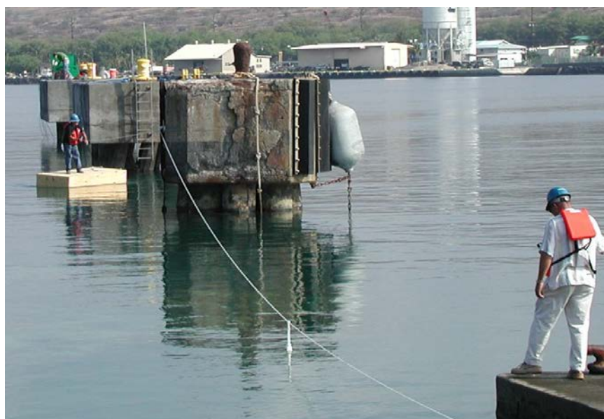
Figure 7. Floating raft used to transport materials and crew.
