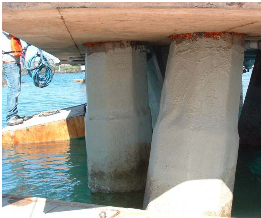
Figure 12. Finished composite wrap assembly.
