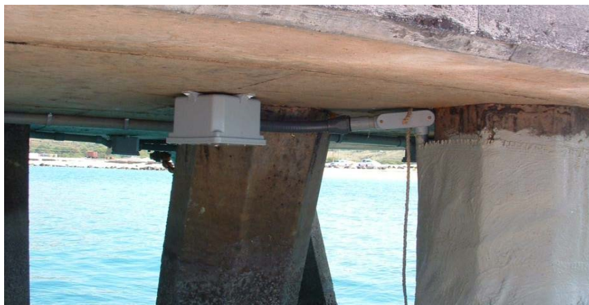
Figure 14. Junction box and conduit attached to underside of pier.
