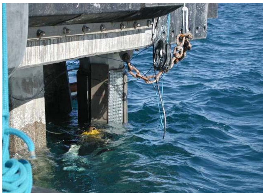
Figure 11. Diver placing compression panel over anode assembly.
