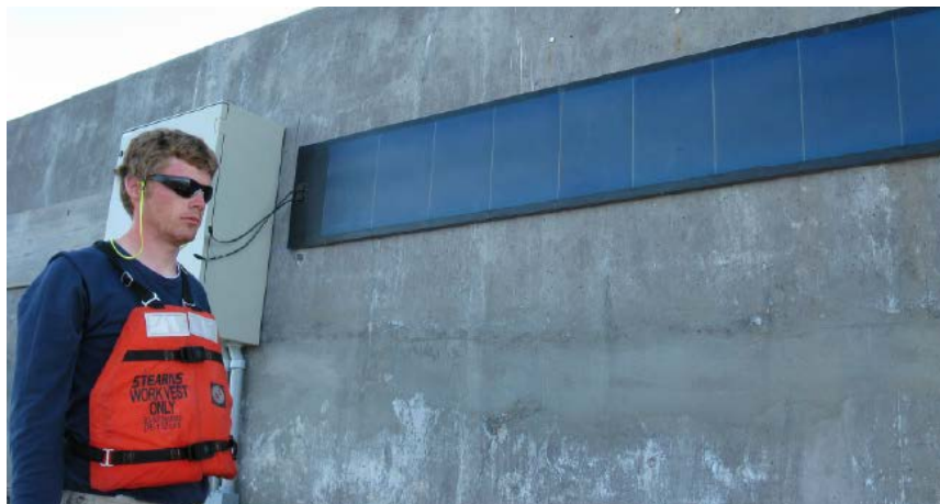
Figure 13. RMU and PV panel mounted on west face of dolphin pier.
