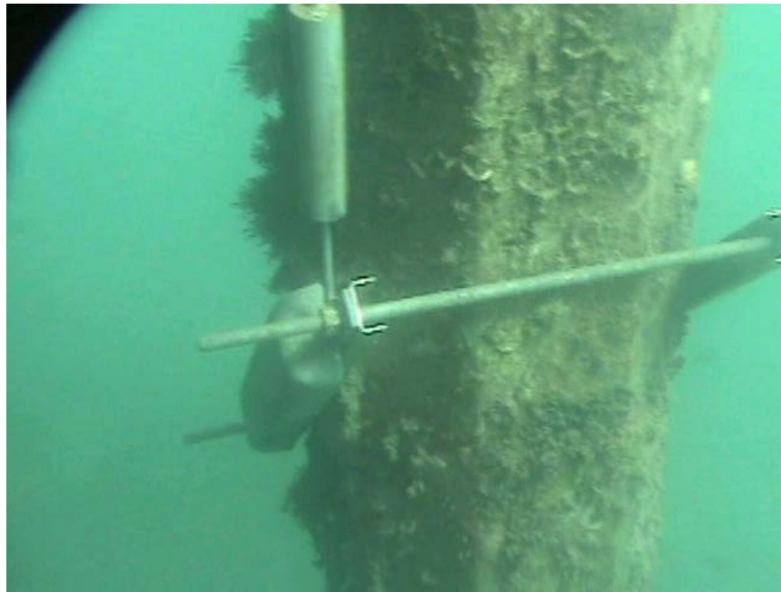
Figure 8. Bulk anode installed at -8.0 MSL elevation.
