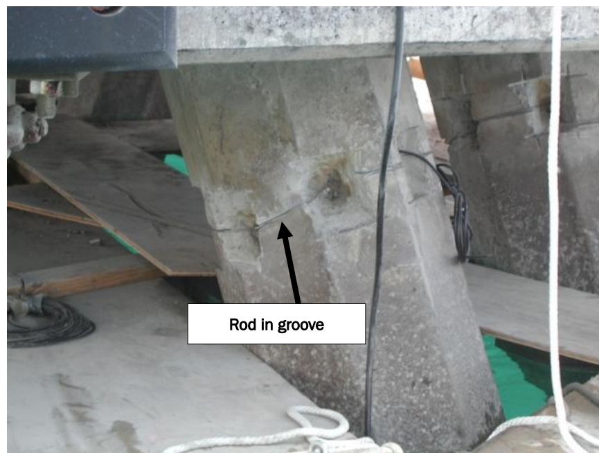
Figure 9. Plugs removed and steel rod placed in grooves.
