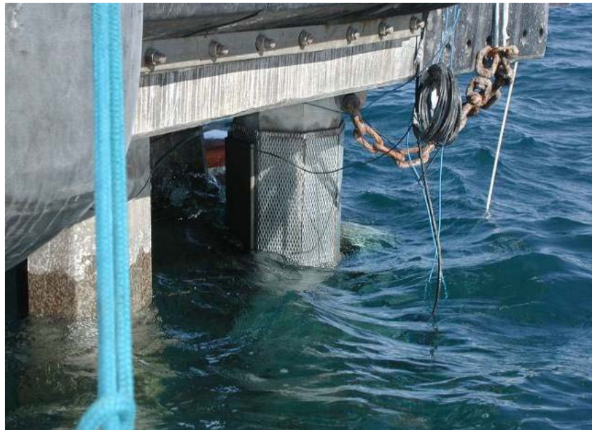
Figure 10. Anode assembly positioned against pile.
