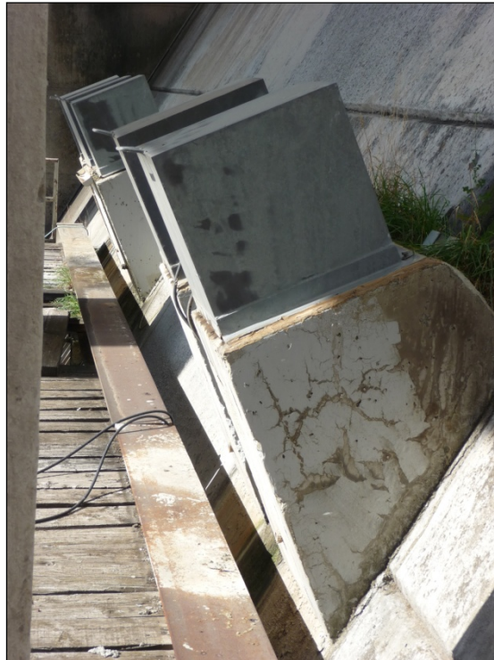
Figure 6-5. Covered anchor head at John Day.
