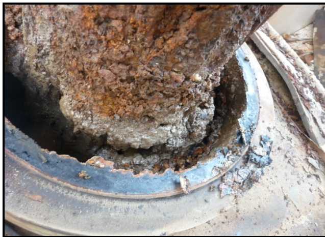
Figure 6-7. Wet grease with rust and possibly mildew contamination (top) and the voided perimeter section (bottom).
