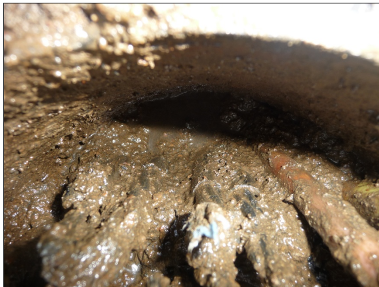
Figure 6-13. No grout detected in anchor heads that were disassembled.
