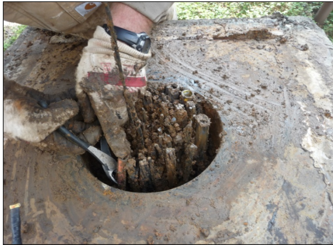
Figure 6-8. Anchor head removed for shipment to ERDC-Vicksburg.
