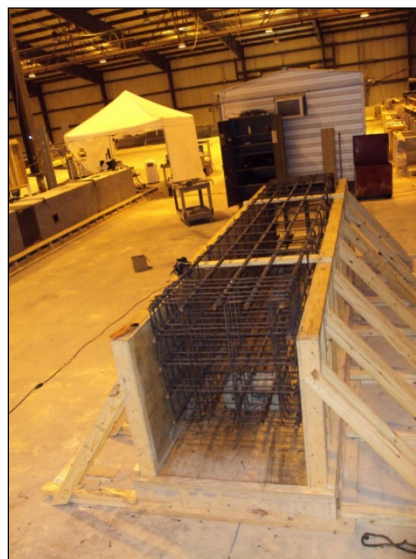
Figure 10-1b. End view of test bed with reinforcement rebar.
