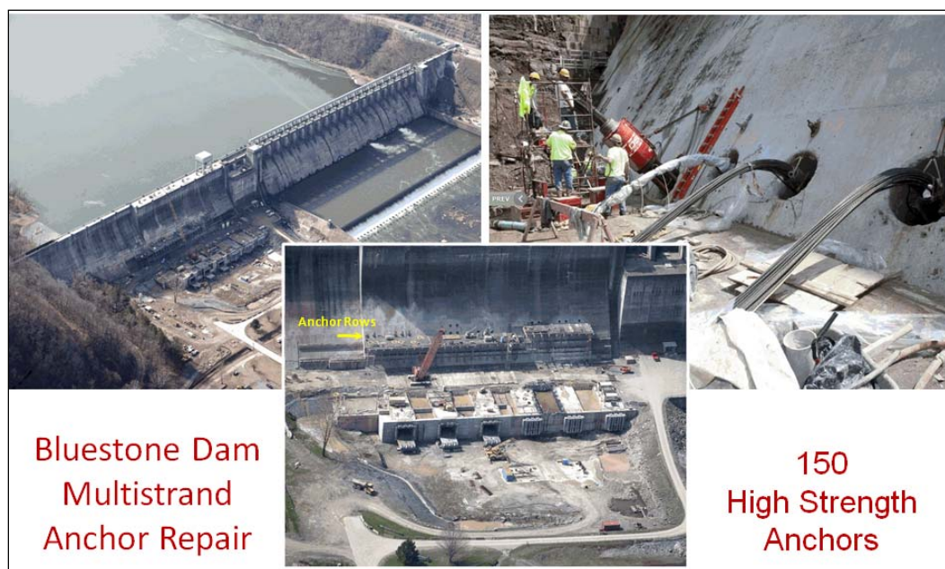
Figure 2-2. Bluestone anchor repair to prevent sliding.
