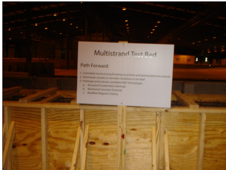
Figure 10-1a. Side view of framing for test bed.
