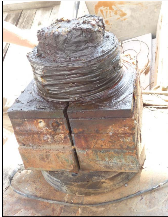
Figure 6-6. Anchor head before removing shim stack.
