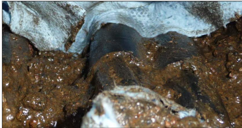
Figure 6-12. Cable sheaths with no signs of deterioration (3/4-in. diameter).
