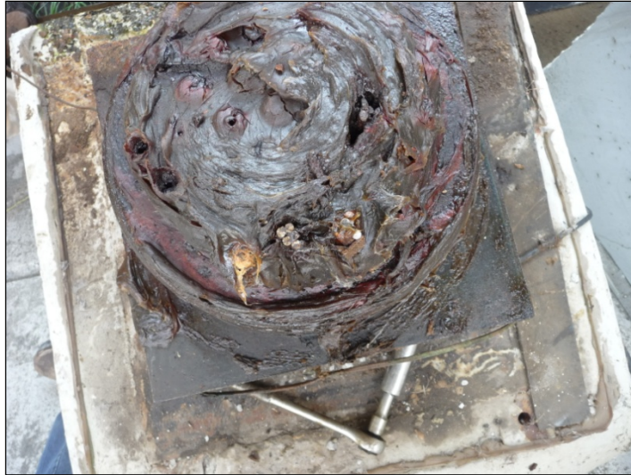
Figure 6-10. Water exits anchor heads through wedges and missing king wires.
