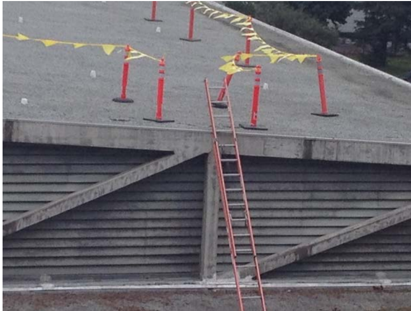
Figure 45. Safety setup at the work area entry point atop King Hall.
