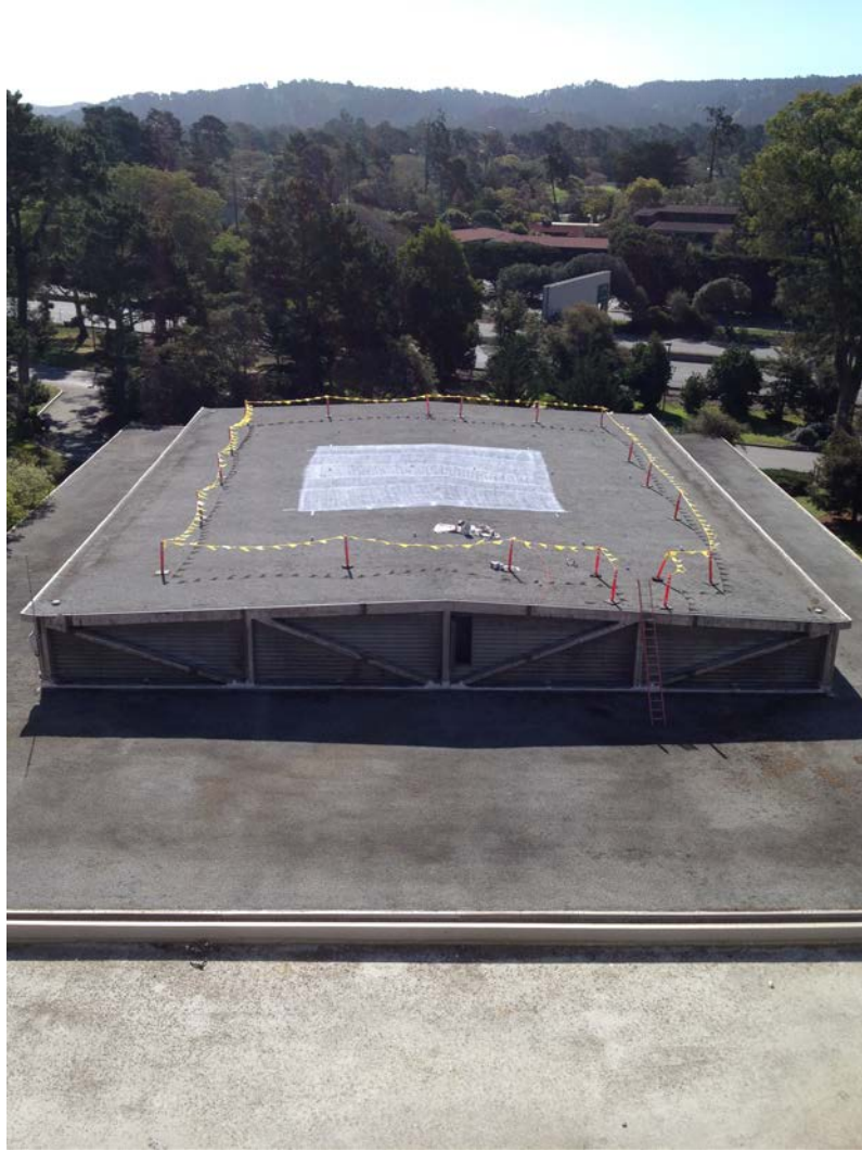
Figure 46. Safety setup atop King Hall showing the complete work area including visual safety barriers and entry point.
