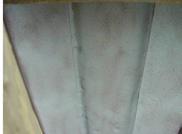
FIGURE 21. Typical appearance of Pensacola SSP just after surface preparation.
