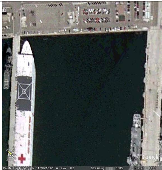
FIGURE 14. Quay wall between Piers 1 and 2, San Diego.
