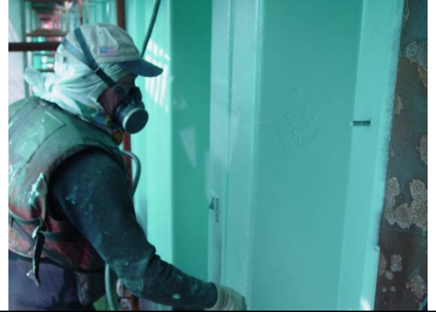
FIGURE 26. Coating Application on San Diego steel sheet piling.
