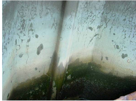
FIGURE 6. PolySpec's Gulf Port field performance at more than one-year service.
