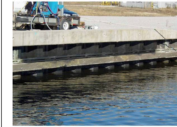
FIGURE 5. PolySpec's Small Scale Installation at Gulf Port, MS.
