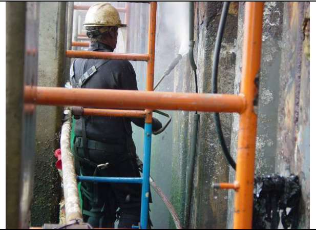
FIGURE 18. San Diego steel sheet pile surface preparation.
