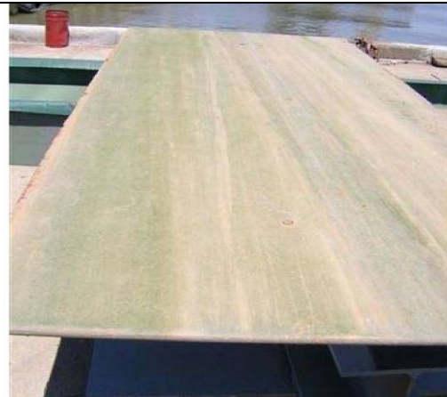
FIGURE 8. Polymeright's CA field performance at more than one-year service.
