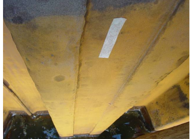
FIGURE 22. Pensacola SSP after flash rusting and before coating application.
