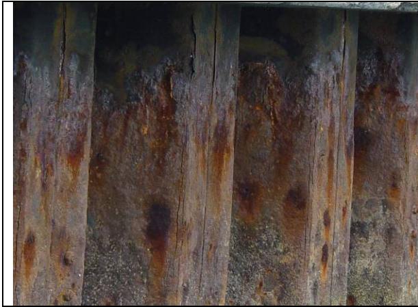
FIGURE 17. Typical corrosion on San Diego steel sheet pile before surface preparation.
