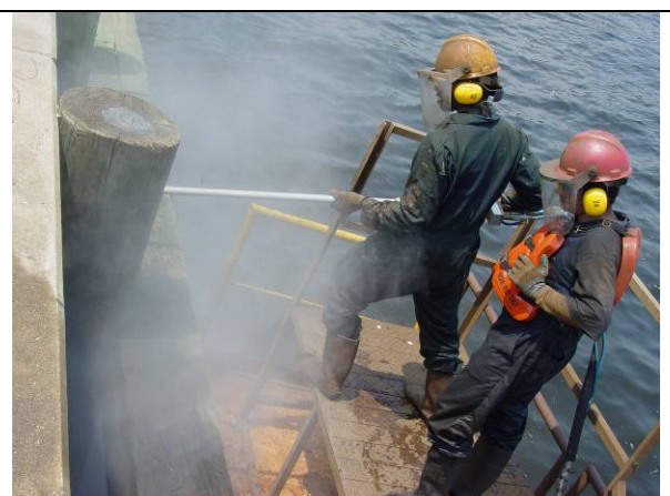
FIGURE 16. Pensacola steel sheet pile surface preparation.
