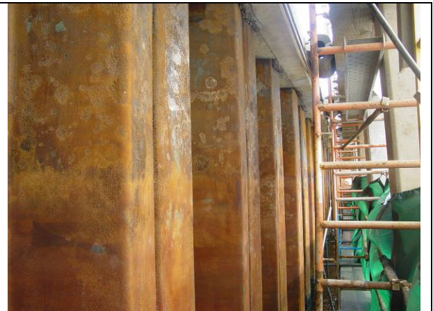
FIGURE 24. San Diego SSP after flash rusting and before coating applications.
