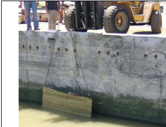
FIGURE 7. Polymeright's Small Scale Installation at San Francisco, CA.
