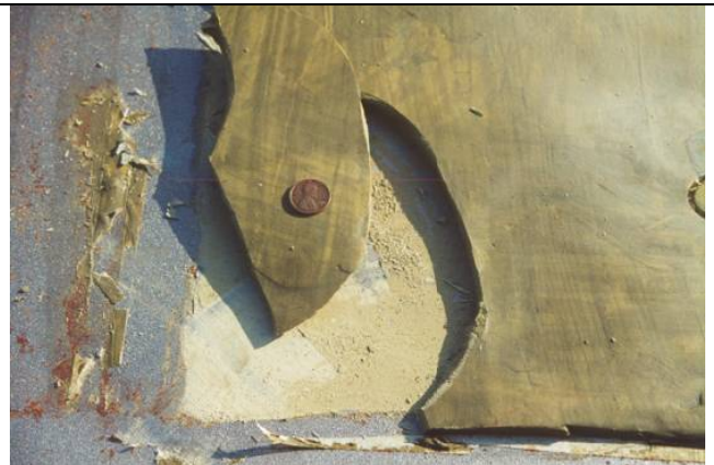
FIGURE 4. Failed Epoxy Putty Adhesion.
