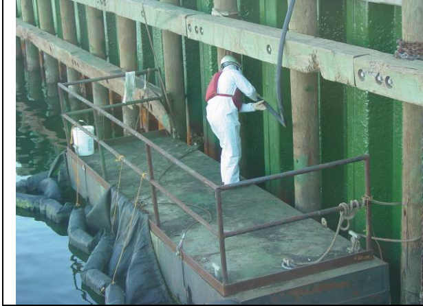
FIGURE 25. Coating Application on Pensacola steel sheet piling.
