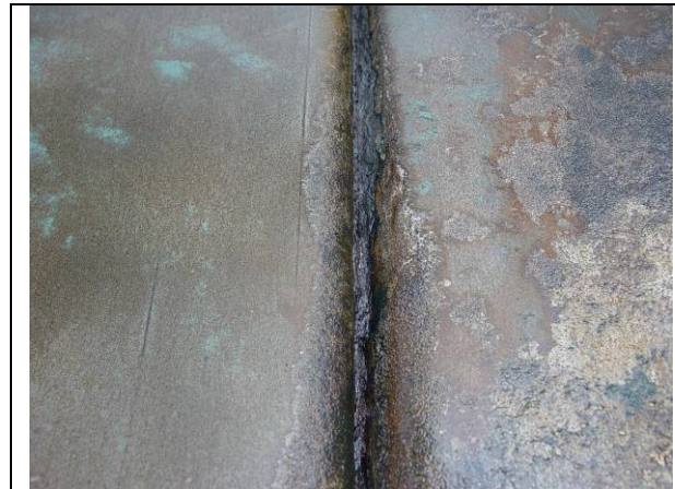
FIGURE 23. Typical appearance of San Diego SSP just after surface preparation.
