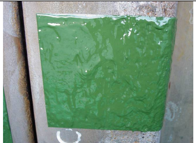
FIGURE 20. Typical test patch – PolySpec coating on San Diego steel sheet pile.
