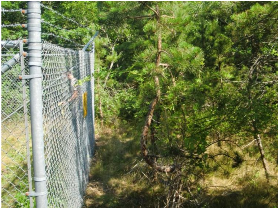
Figure 6.4. LF-7 Site, South Side Exterior Fence and Radioactive Markings
