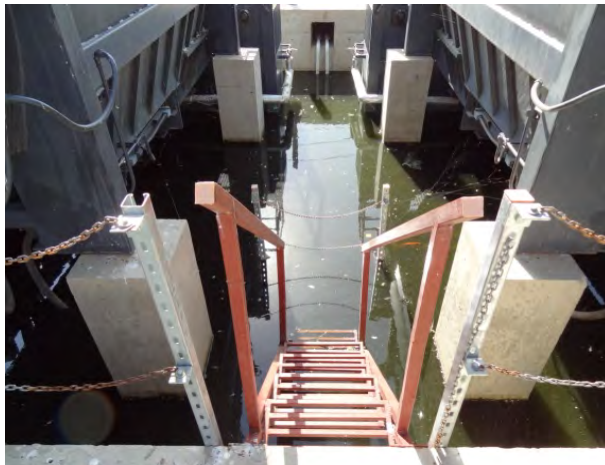
Photo 3 - Stagnant Water in Bilge Pit Beneath Incinerators
