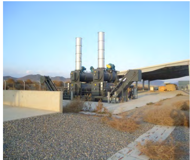
Photo 1 - Two 8-Ton Capacity Incinerators at FOB Salerno
