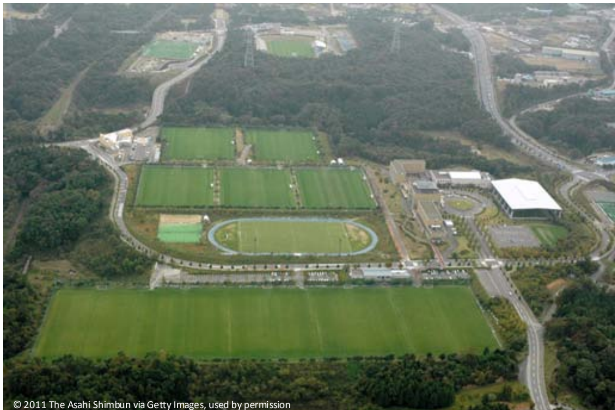
Figure 1. Aerial view of the J-Village complex (looking south)
