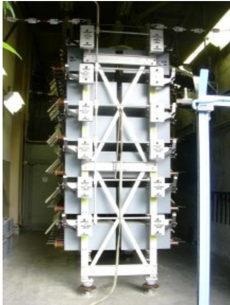
Figure 4: 1.2 MJ capacitor bank.
